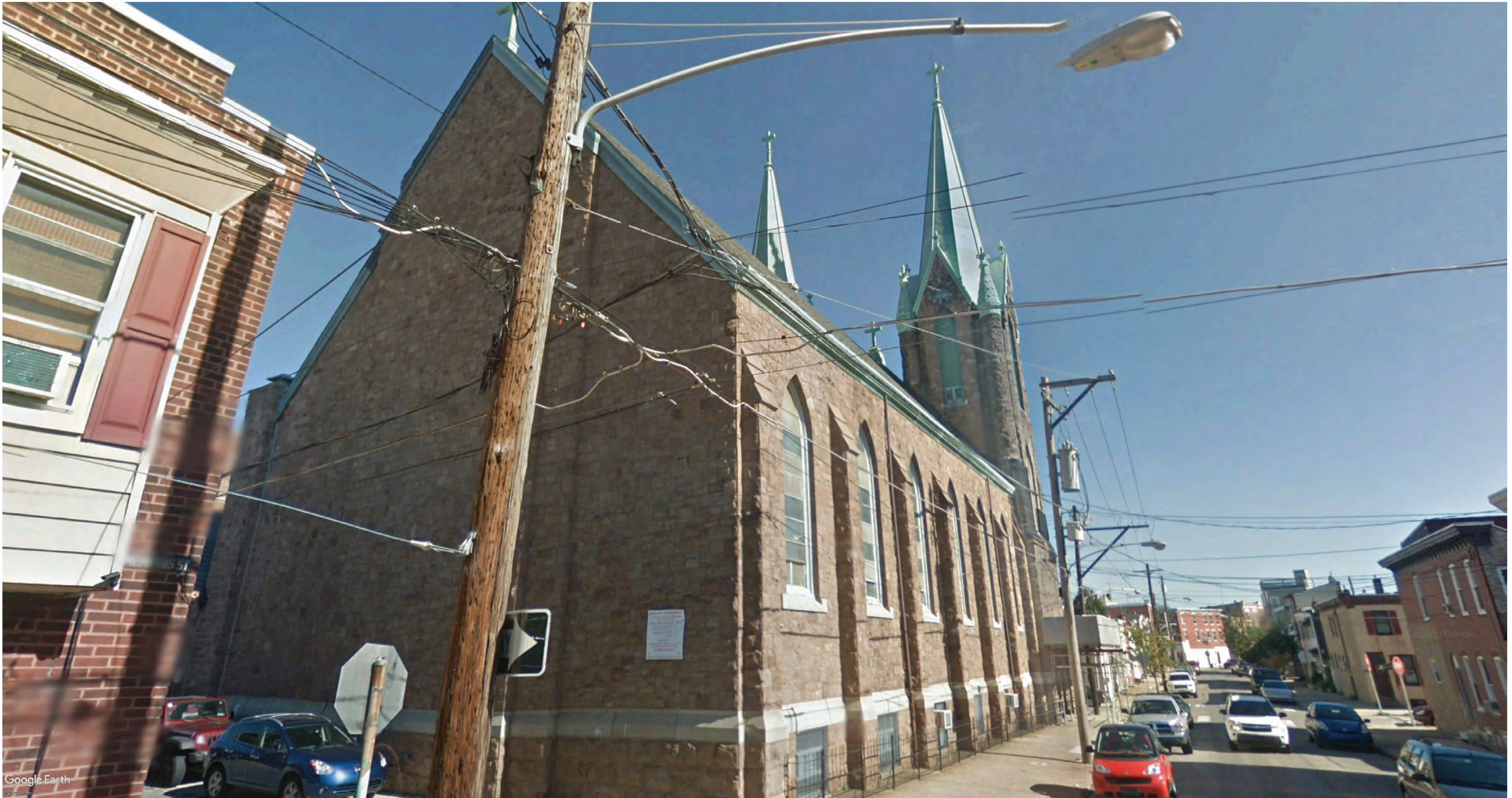
BERKS ST TOWNHOMES SITE - PREVIOUS CATHEDRAL UNDER DEMOLITION | BERKS & MEMPHIS
