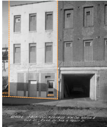
IMAGE 4 - (1953) FACADES ALONG N. WATER STREET
