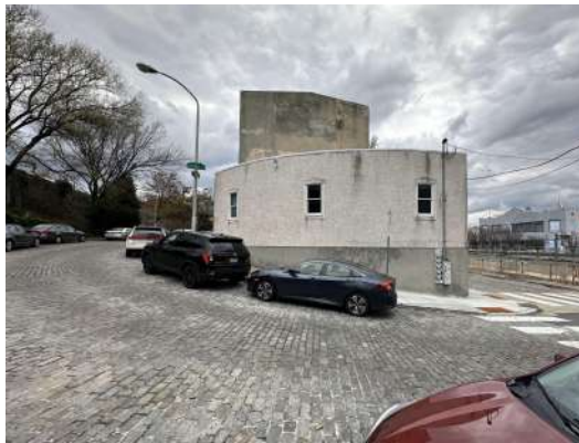
IMAGE 7 - (2024) VIEW NORTHWARD FROM VINE STREET
