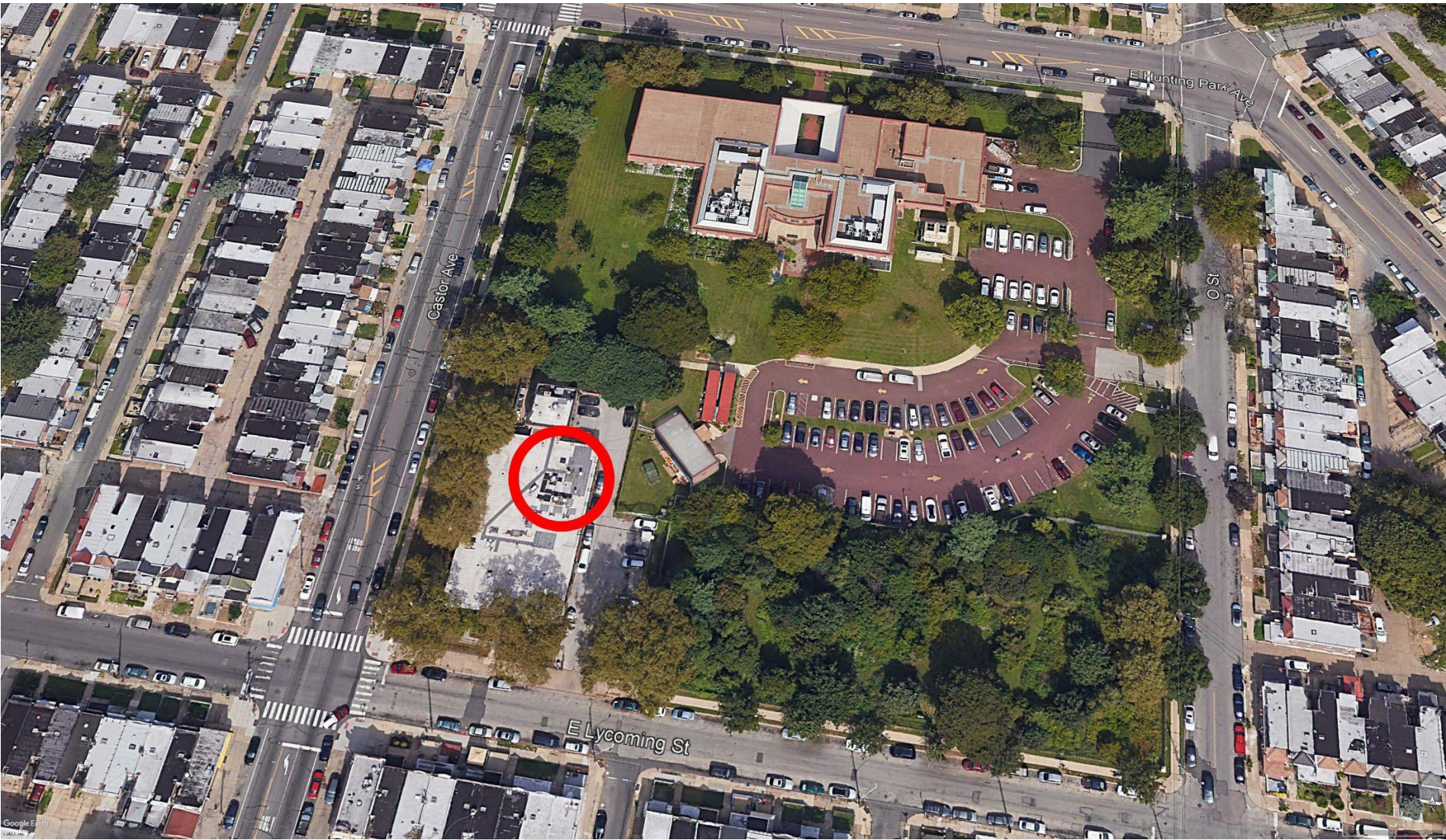
Figure 3 – LAB North Aerial View
