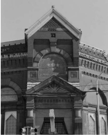
Figure 27. Northwestern National Bank, 1828 Girard Avenue (HABS report, 2000).
