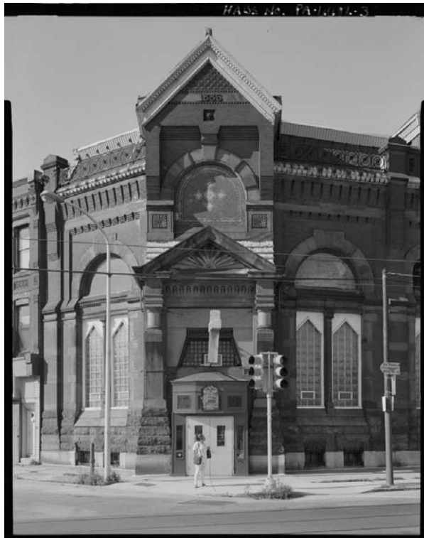
Figure 13. Northwestern National Bank building at Ridge Avenue and Girard Avenue constructed 1886-87.
