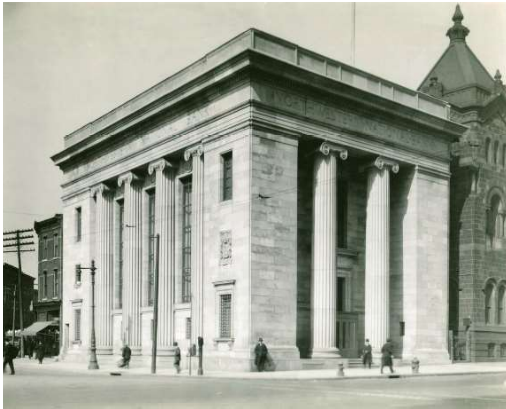
Figure 15. Northwestern National Bank building with construction nearing completion in 1918. Bank signage and lighting have not yet been installed (Indiana University Bloomington, Indiana Limestone Photograph Collection).
