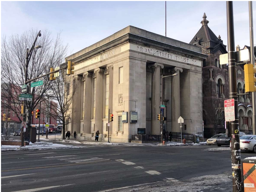
Figure 13. View of 700-02 N Broad Street at the corner of N Broad Street and Fairmount Avenue.
