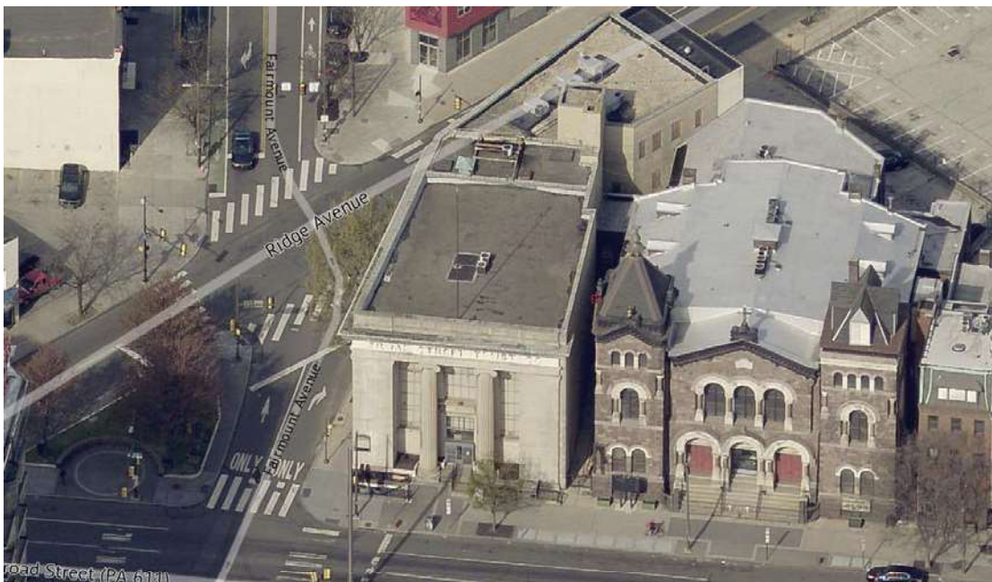
Figure 12. Aerial view looking northwest. This view shows the original rectangular front section of the building. The addition is shown at an angle off of the rear of the original building. The north elevation walls, in between 700-02 N Broad Street and the adjacent church, are clad in buff colored brick (image from CONNECTExplorer ).
