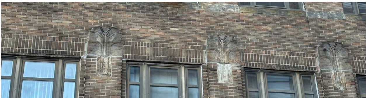
Figure 7. Detail of brick pilasters with stylized chevron sandstone caps, March 2025.
