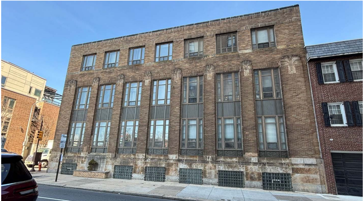
Figure 6. Lombard Street elevation, March 2025.
