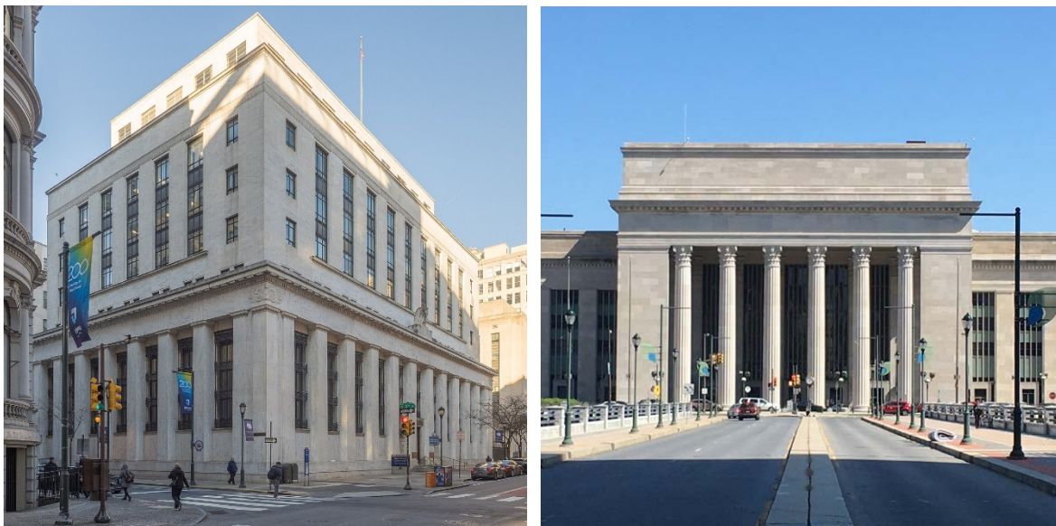
Figure 17: Left: Old Federal Reserve Bank Building, image courtesy Wikimedia Commons. Right: William H. Gray III 30 th St. Station, image courtesy Amtrak.
