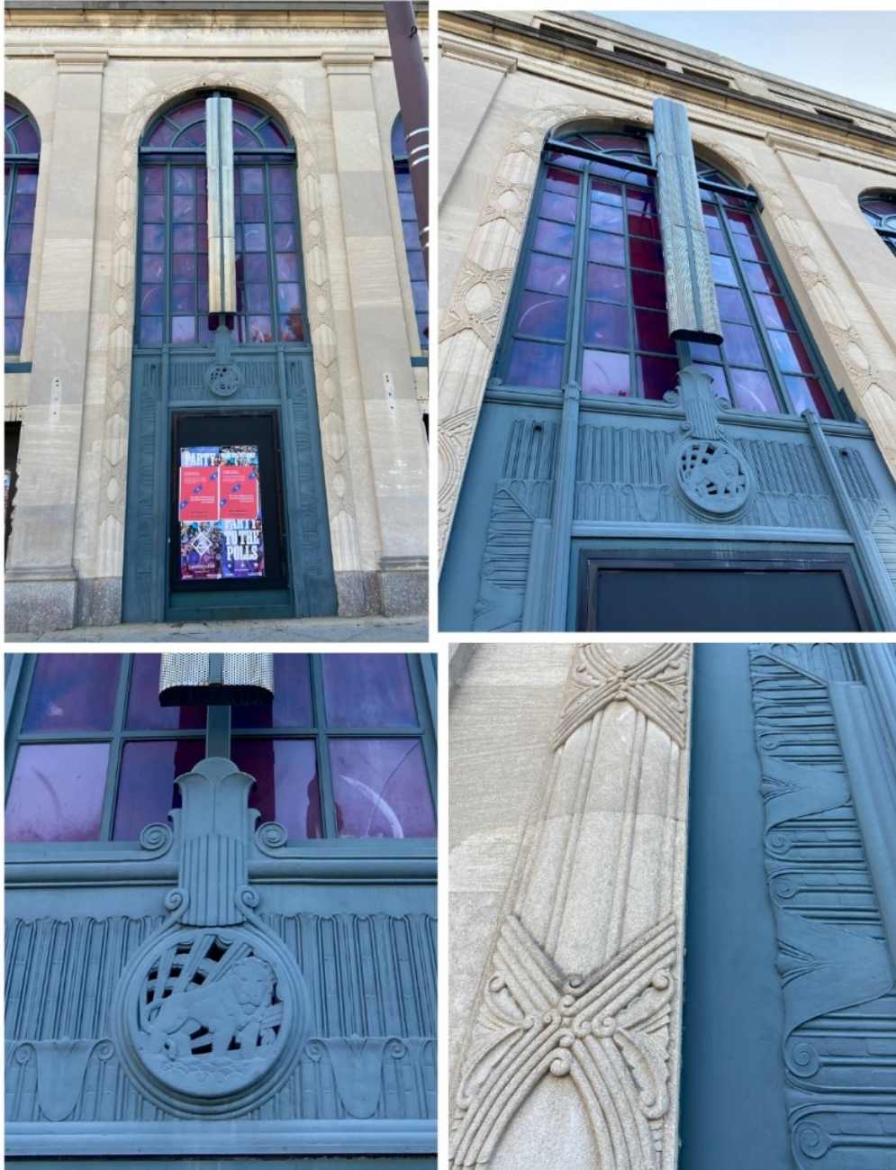
Figure 4. Centermost bay of the façade.
