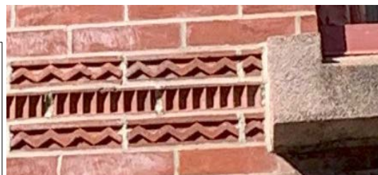
Figures 18, 19, and 20: The lower decorative belt course, which uses No. 179 and No. 182 from the 1890 Peerless catalog.
