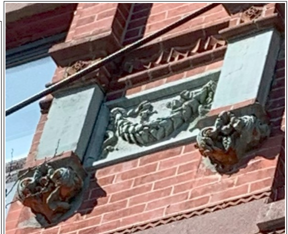
Figures 39 and 40: A protruding course of somewhat deteriorated notched brick, style 135, aligns with a notched band that echoes the design of the parapet wall cornice behind it. Two pairs of sloped panels (the larger one incised with a curved decoration) soften the transition between setbacks.
