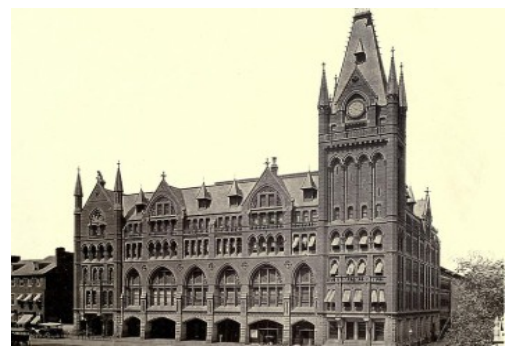
Figure 104: Broad Street Station, Penna RR, Wilson Brothers & Co, 1885
