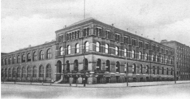
Figure 101: Office of Baldwin Locomotive works, Wilson Brothers & Co, 1900.
