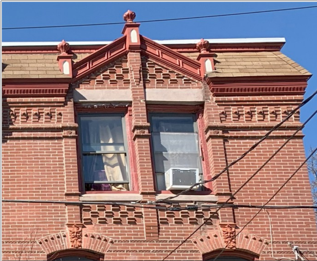
Figure 21: The third floor of 1631 Francis St.
