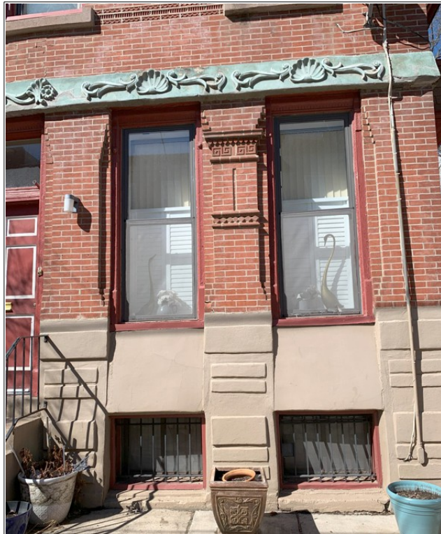
Figure 5: The first floor of 1631 Francis St.
