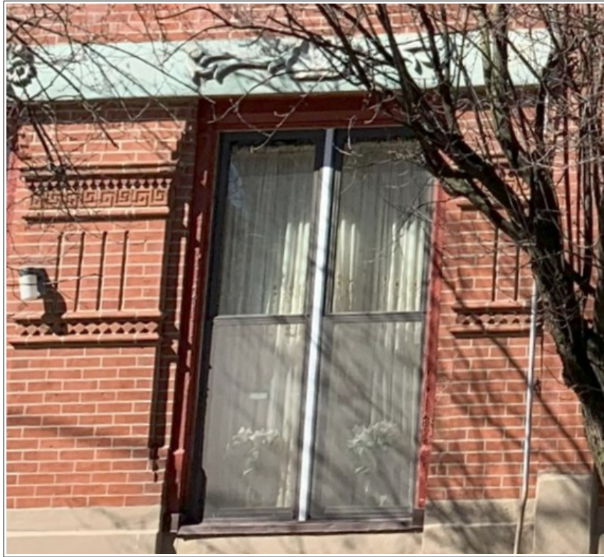
Figure 49: The first-floor windows of 1635 Francis St.
