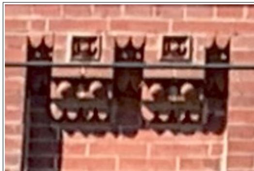
Figure 38: Under the pediment, below two courses of plain brick, are a pair of ornaments assembled in a novel way from molded bricks (style 10, 144, and 288) used elsewhere on the facade.
