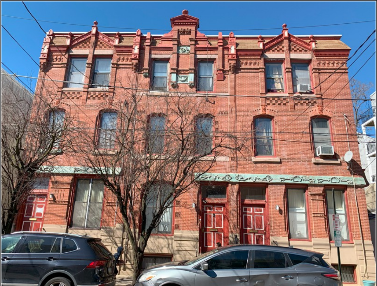
Figure 4: Right to left: 1631, 1633, and 1635 Francis Street, looking northwest.
