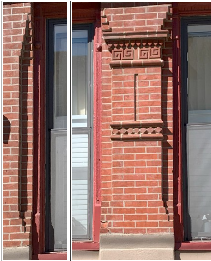
Figures 7 and 8: Detail of brickwork around windows.
