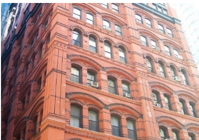
Figure 94: Morse Building, New York City, Silliman and Farnsworth, 1880.
