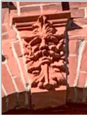
Figures 15, 16, and 17: The second-floor windows feature decorative arches using Peerless brick No. 10 and topped with a Green Man keystone.
