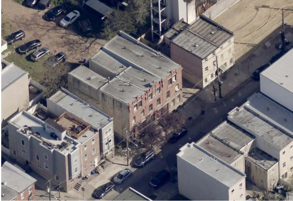
Figure 2: The properties sit at the corner of Francis St and Field St.
