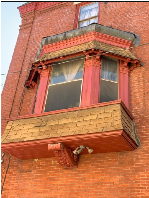
Figures 27 and 28: Details of the oriel window and its supporting bracket.
