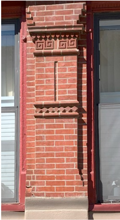
Figure 4: Detail of 1631 Francis St and corresponding decorative bricks from Peerless Brick Company's 1890 catalogue.
