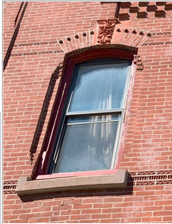
Figures 15, 16, and 17: The second-floor windows feature decorative arches using Peerless brick No. 10 and topped with a Green Man keystone.
