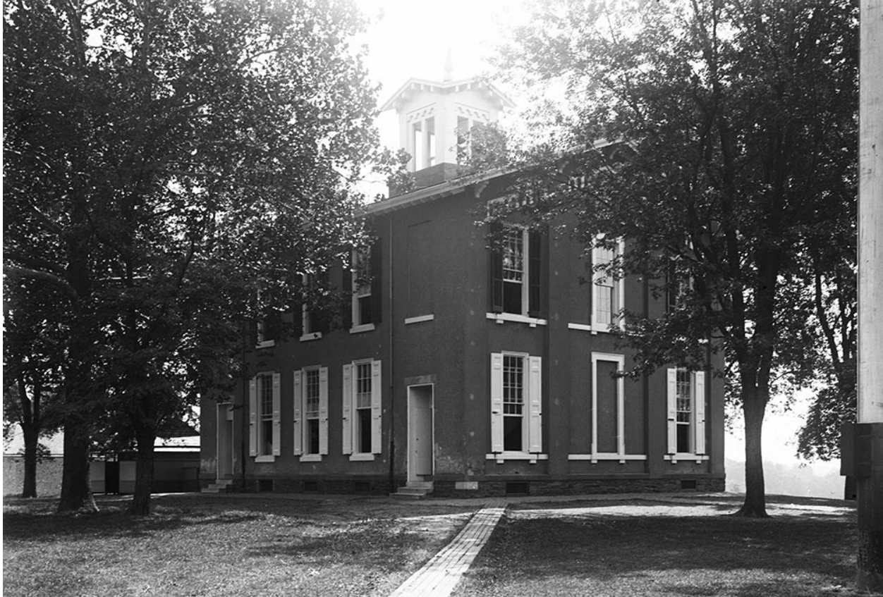
Figure 20. The Fayette Public School, Samuel Sloan, architect, 1854; photograph by Franklin Davenport Edmunds, September 10, 1912. (Source: Free Library of Philadelphia)
