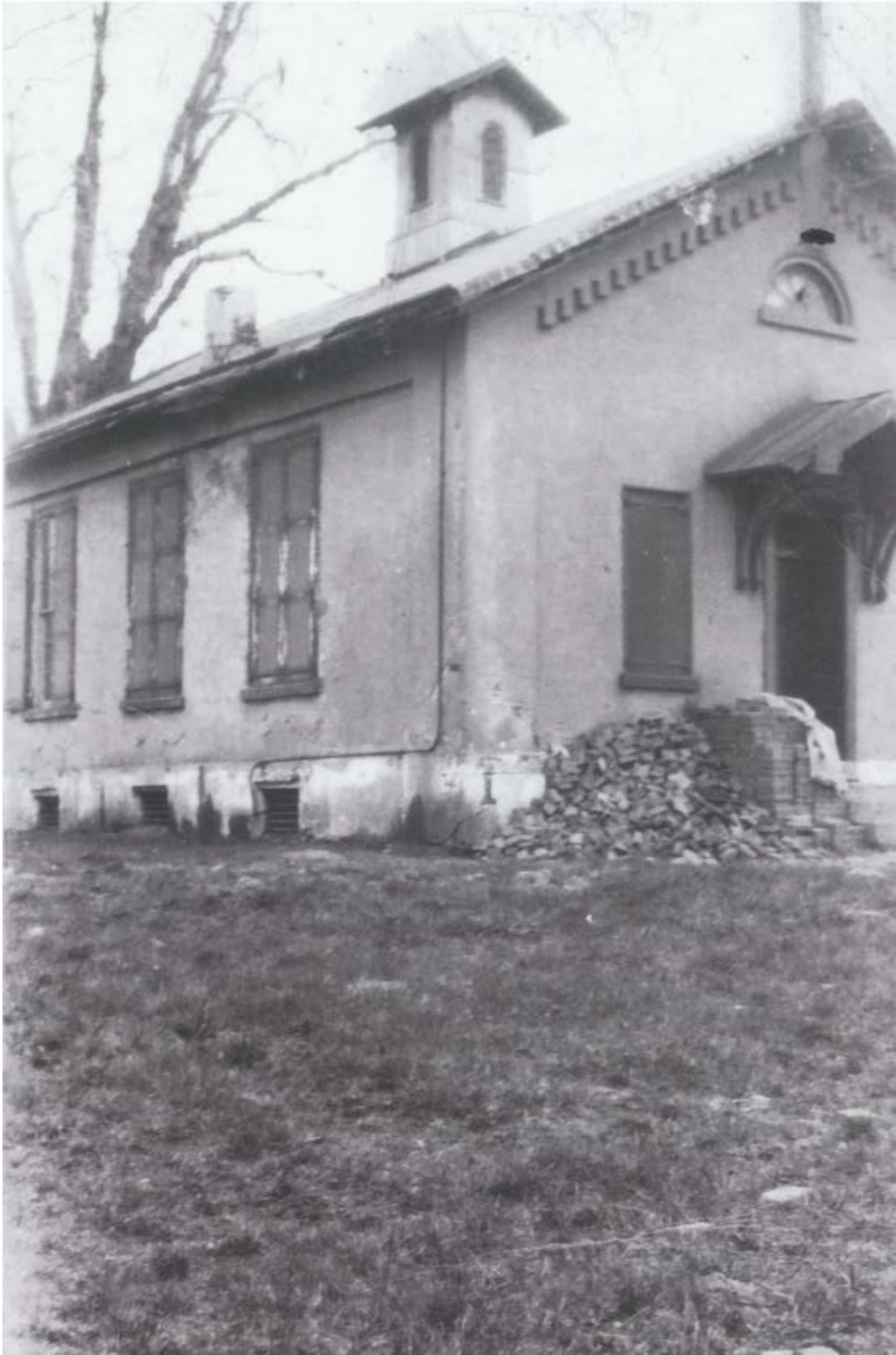
Figure 1. Front (north) and side (east) facades of the Maple Grove School, 10151 Academy Road, 1936, prior to conversion from schoolhouse to dwelling.
