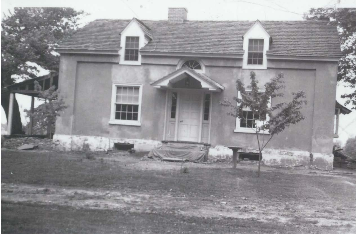
Figure 5. Side (west) facade of the Maple Grove School, 10151 Academy Road, 1939, after conversion from schoolhouse to dwelling. The canopy over the doorway and the lunette window were moved from the front façade to this façade. The first-floor windows were shortened and the dormers were added.
