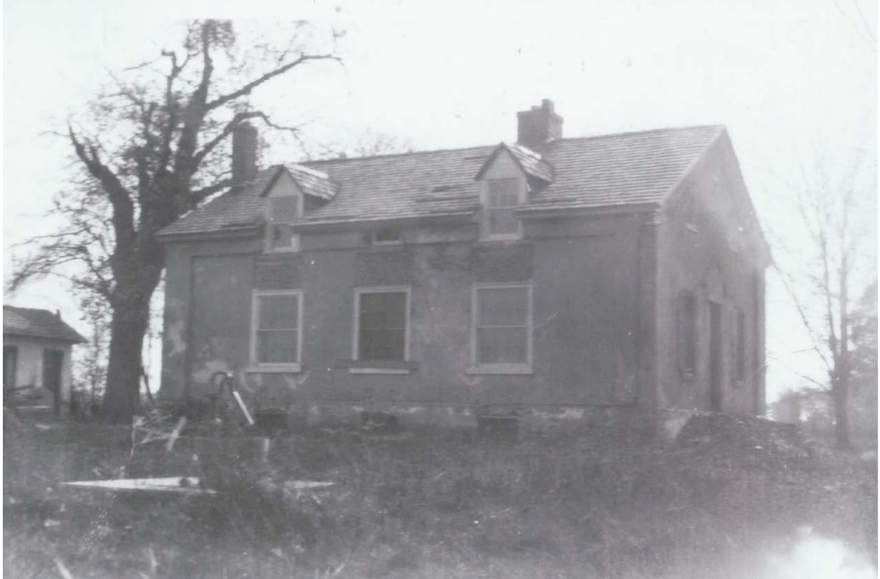
Figure 6. Side (east) facade of the Maple Grove School, 10151 Academy Road, 1939, after conversion from schoolhouse to dwelling. The first-floor windows were shortened and the dormers were added. The school outhouse can be seen to the left by the tree.
