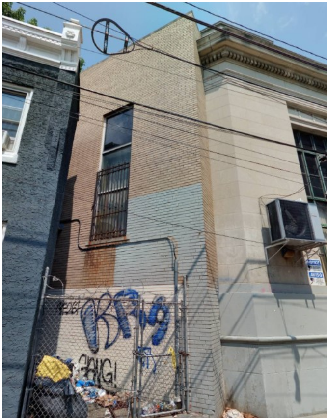
Figure 4. South facade of 820-26 E Allegheny Avenue, (Partial) August 2024. Source: Cyclomedia.
