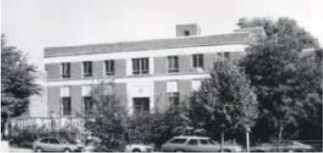
Figure 57. Manhattanville College Library, Paul Monaghan, Architect, 1941. Demolished. Source: Buildings of City College, slideshare.net.
