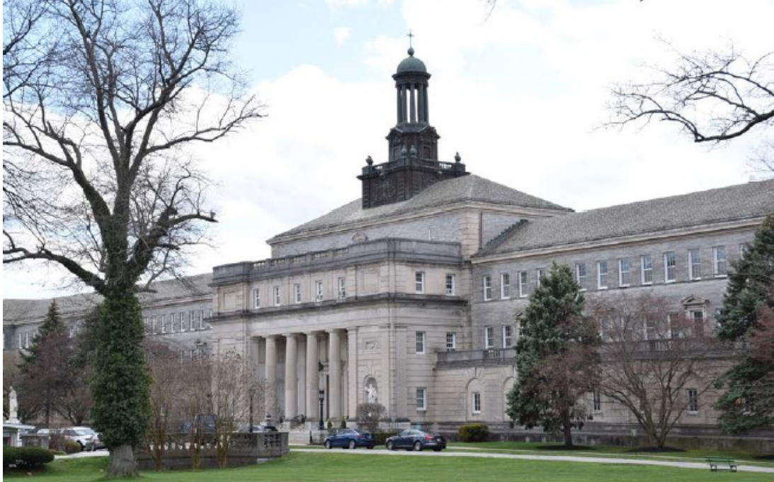
Figure 50. St. Charles Borromeo Seminary, Detail. Paul Monaghan, Architect, 1928 Source: Determination of Eligibility for St. Charles Borromeo Seminary, 2023. Source: PA Share.
