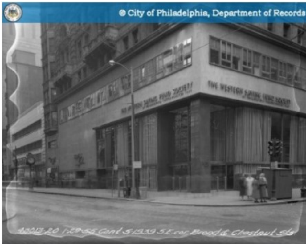
Figure 27. WSFS Bank Renovation. Source: City of Philadelphia, Department of Records, 1955.
