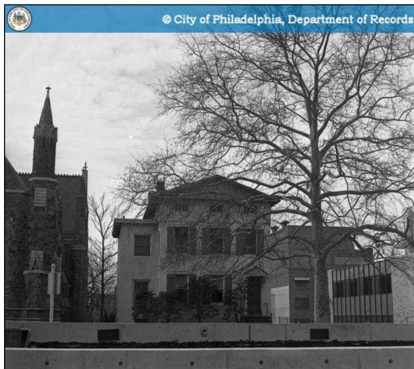
Fig. 12. Photograph dated 1971 showing window shutters at north elevation. Source: City of Philadelphia, Department of Records.
