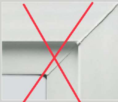
Typical welded vinyl corner seam with distracting ridges
