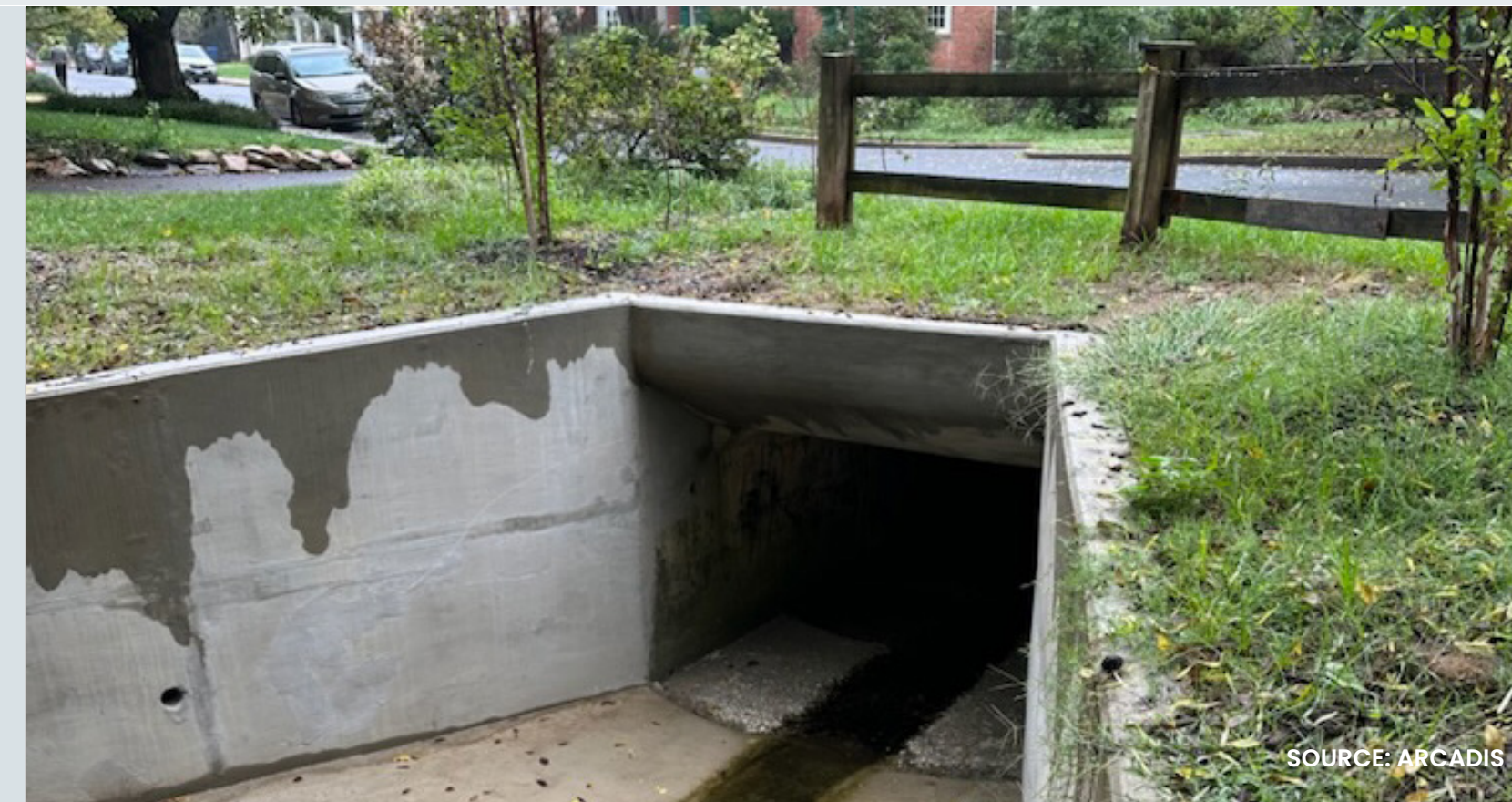
EXAMPLE OF ENLARGED PIPES AND CULVERTS
