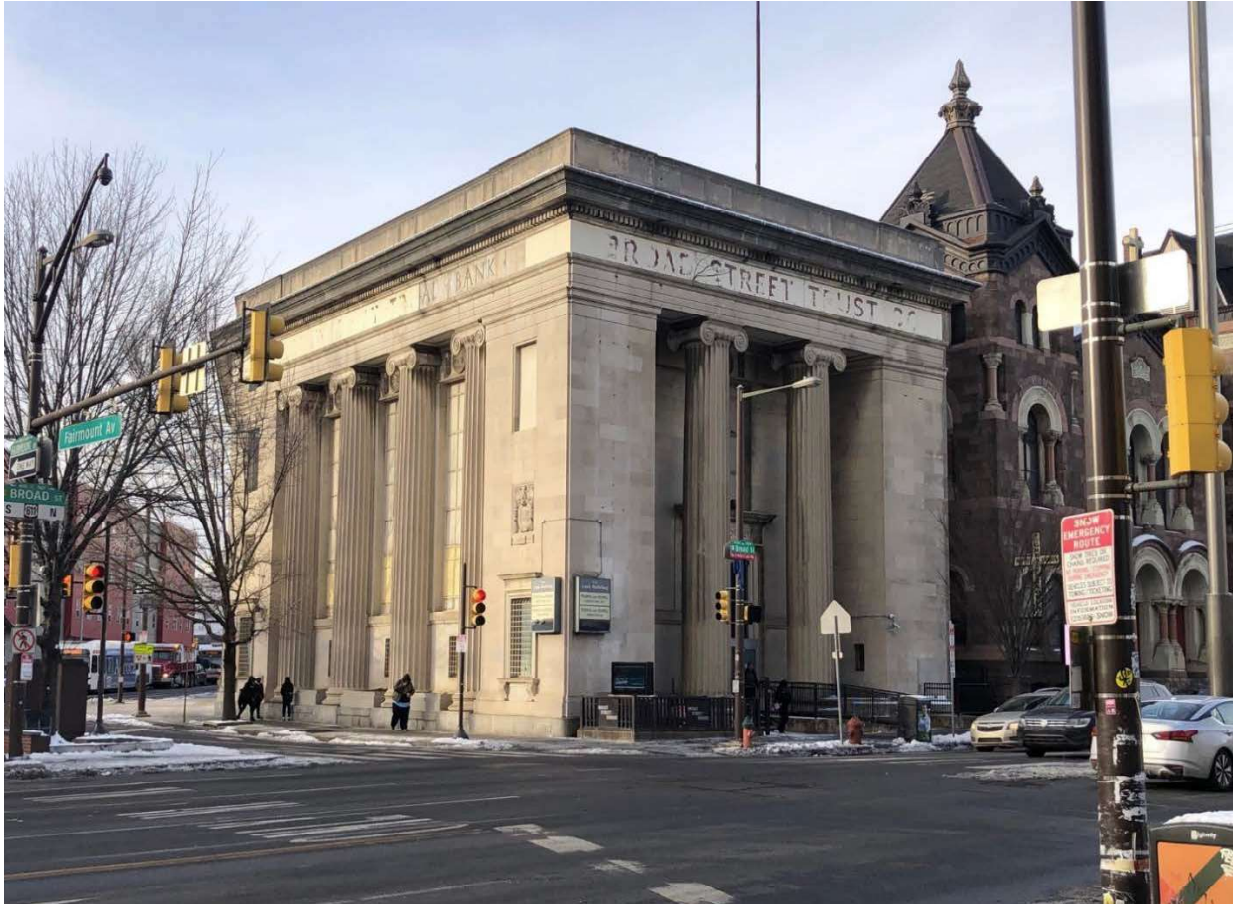
Figure 4. A view of the corner of Broad Street and Fairmount Avenue showing the original section of the building constructed in 1917-18.
