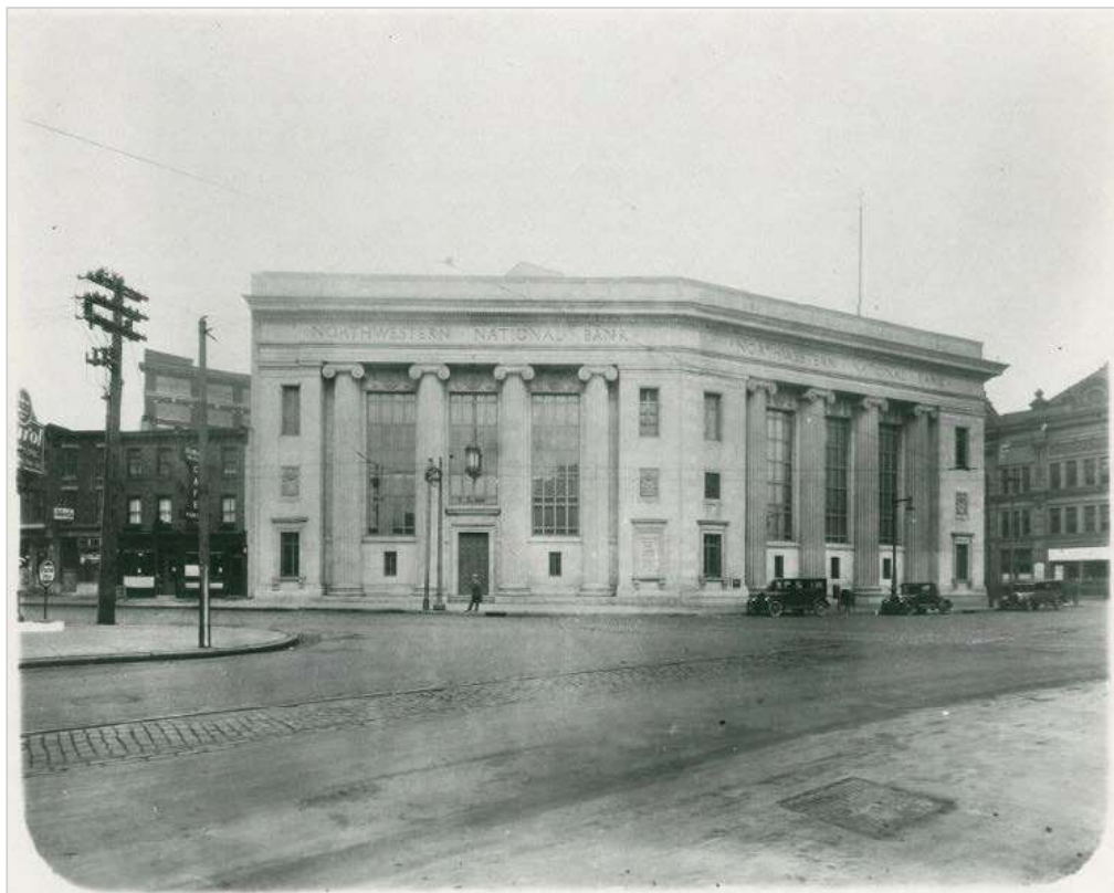
Figure 2, top image. Circa 1920. Early photograph shows the original rectangular form of the building located at N Broad Street and Fairmount Avenue (Indiana University Bloomington, Indiana Limestone Photograph Collection). Figure 3, lower image. Circa 1930. This photograph was taken after the addition was constructed in 1929. The addition (on left side of image with man standing in front of entrance) doubled the size of the building. (Jacob Stelman Collection, Athenaeum of Philadelphia).
