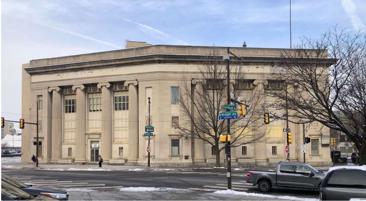
Figure 7. View of the elevations along Ridge and Fairmount Avenues. The section along Ridge Avenue was added in 1929 and faithfully replicated the architecture, materials, and craftsmanship of the original building. The addition created a secondary entrance to the bank.
