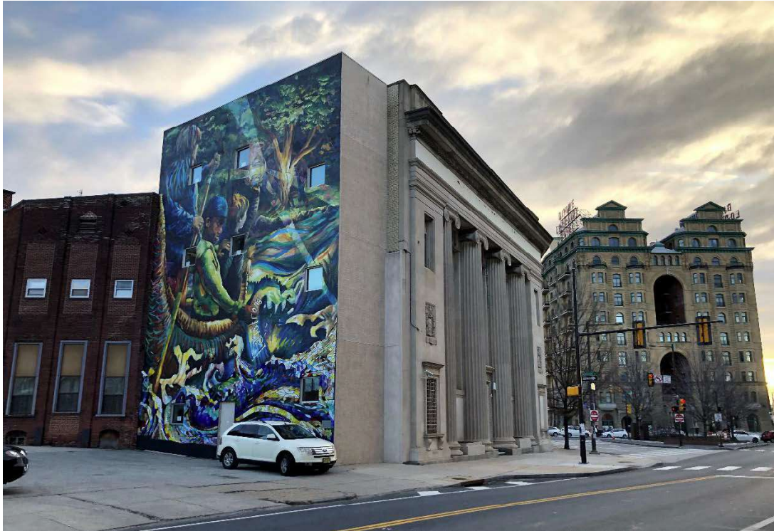
Figure 11. View of the rear of building. A parking lot is located behind the building. In 2008, an enclosed fire/exit stair has been added to the rear of the building along Ridge Avenue. It is clad in stucco and the rear wall displays a painted mural.
