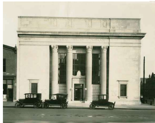
Figure 32. Federal Trust Company, South Broad and Federal Streets, extant.
