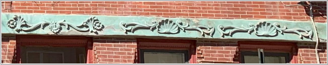
Figure 14: A decorative band of stone runs above the first-floor windows and door.
