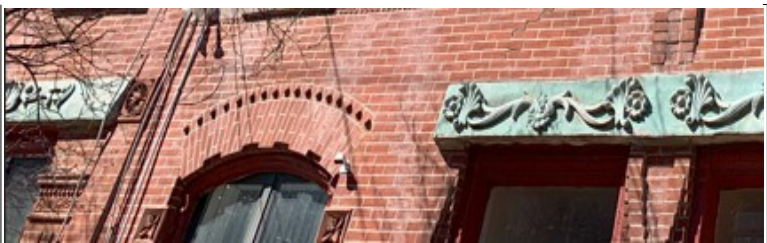
Figure 34: Notably, the arch interrupts the stone band course that otherwise runs the entire width of the three properties.
