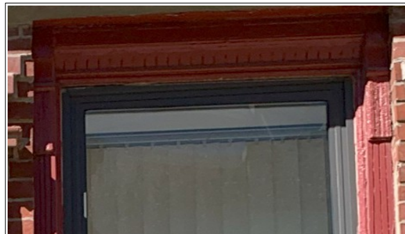
Figure 6: Detail showing the decorative trim around the transom.
