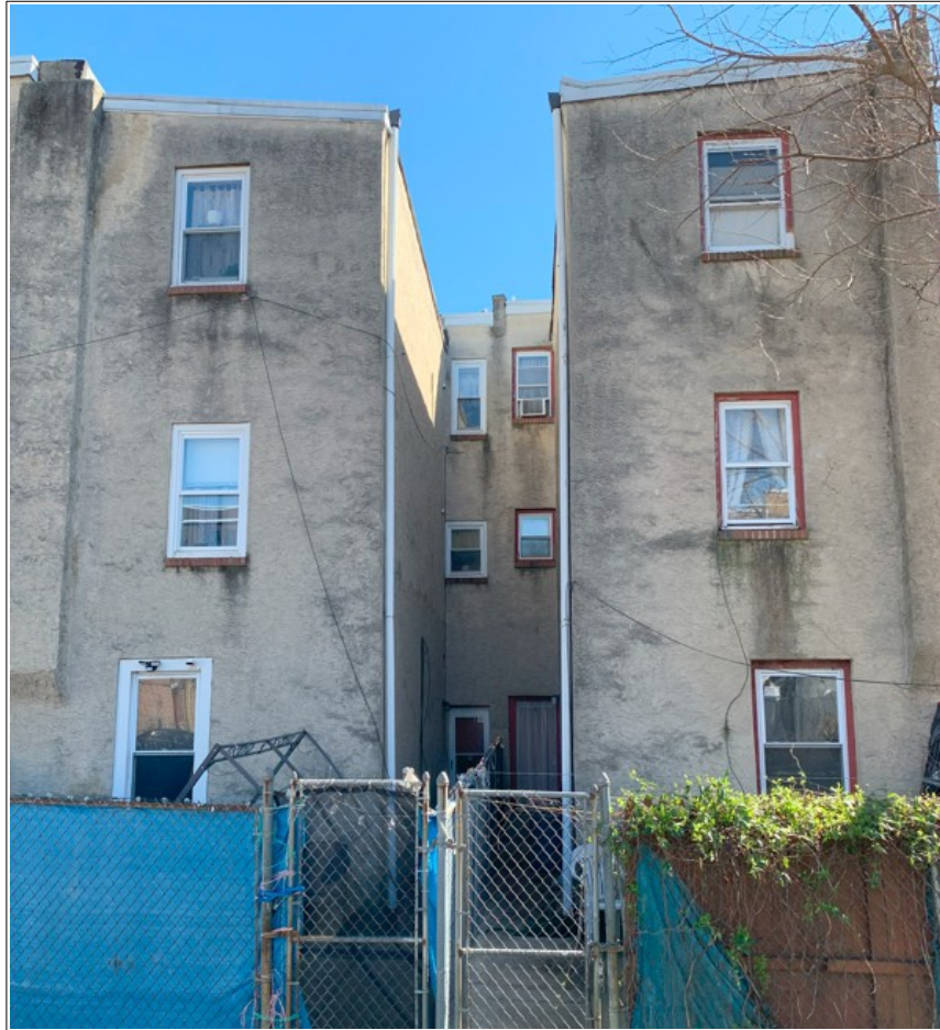
Figure 48: Rear elevations of 1633 (left) and 1635 (right) Francis Street, looking southeast.
