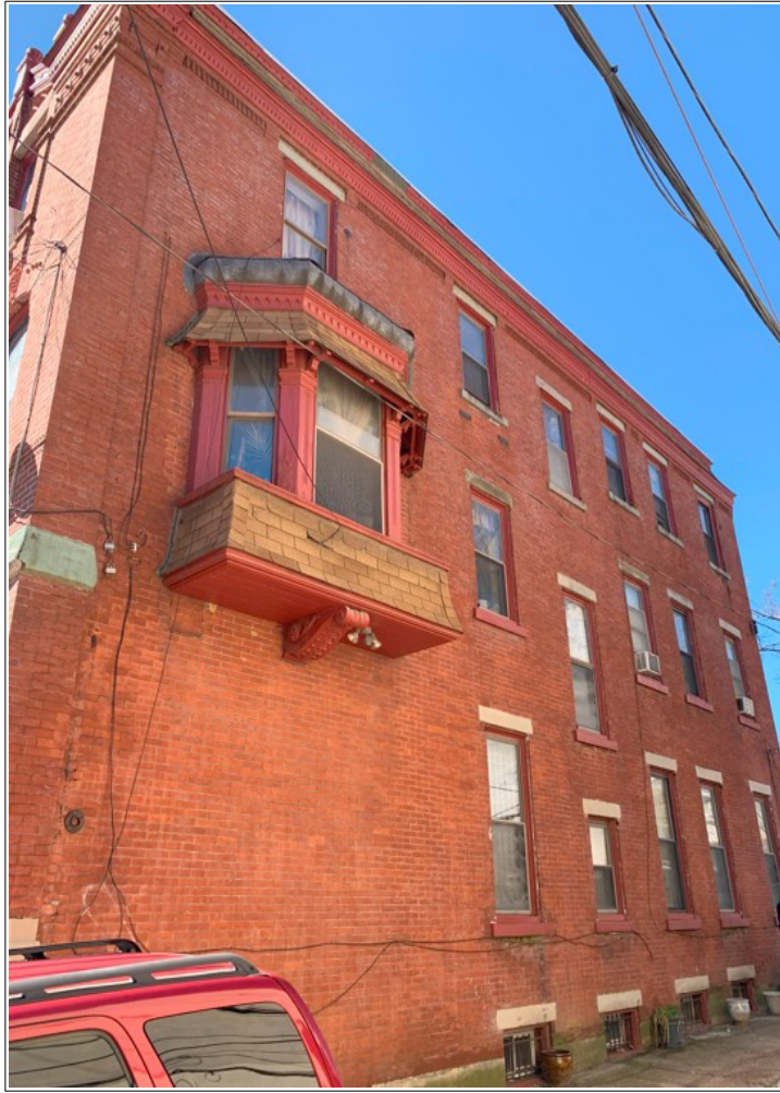
Figure 26: The Field St elevation, looking west.
