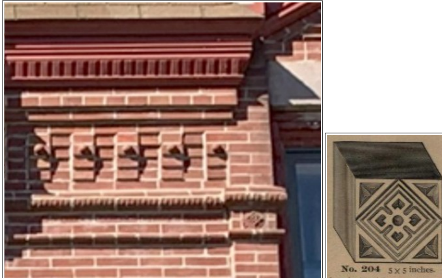
Figures 24 and 25: Detail showing ornamental brick bands and cornice.
