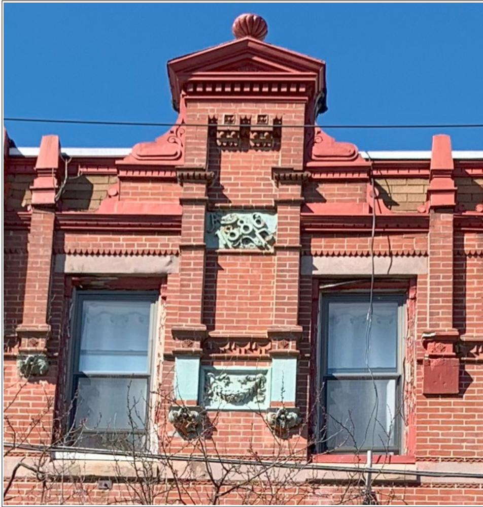
Figure 37: Extensive ornament at the top of the façade of 1633 Francis St serves as a central element for the three adjoining properties.
