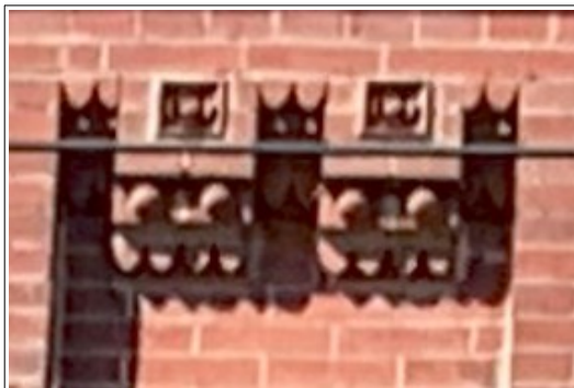
Figure 38: Under the pediment, below two courses of plain brick, are a pair of ornaments assembled in a novel way from molded bricks (style 10, 144, and 288) used elsewhere on the facade.
