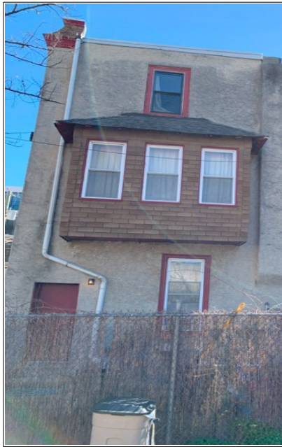
Figure 31: Rear elevation of 1631 Francis St, looking southwest.
