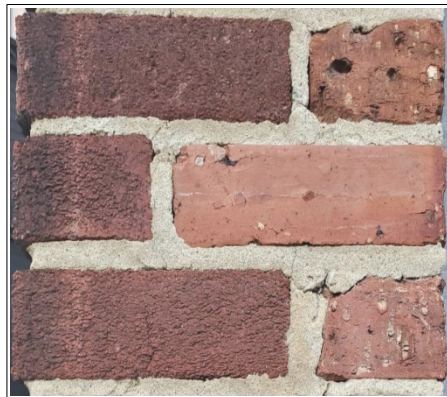
Figure 68: Both pressed brick and common brick are visible in this photo from a building in Washington, DC. The pressed brick (darker, left) is more uniform, while common brick (lighter, right) has more variation and visible particles of stone.
