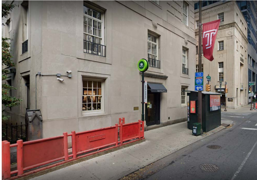
1601 Locust St. with its two raised ground-floor windows
