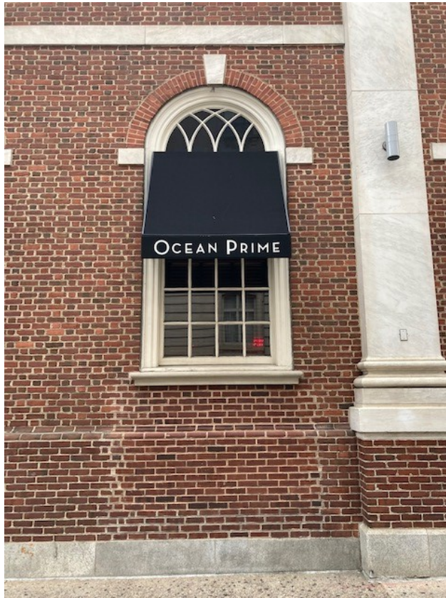
130 S. 15 TH STREET. DETAIL OF CLOSED UP WINDOW OPENING SHOWING SCARRING FROM REVERSED ENLARGEMENT. PHOTO BY PAUL STEINKE, 8/17/21.
