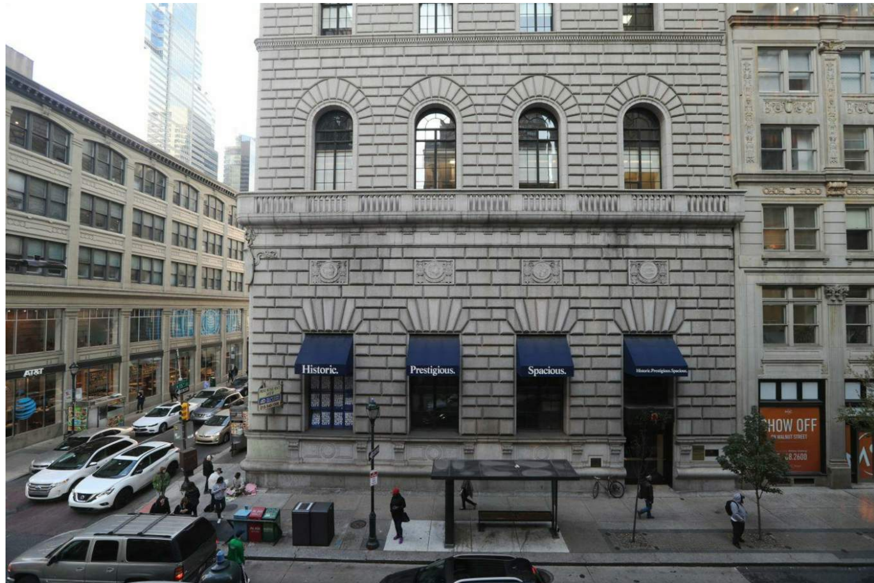
4 WALNUT STREET FACADE
