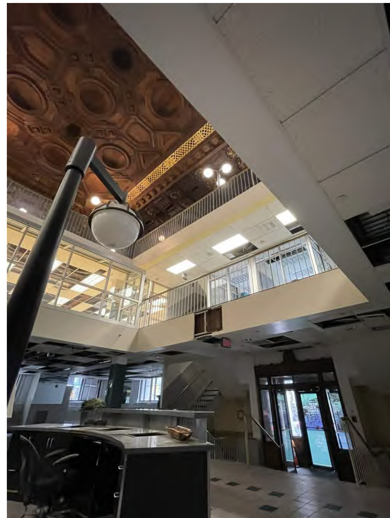
5 15TH STREET ENTRANCE WITH EXISTING MEZZANINES INTERIOR VIEW FROM FIRST FLOOR (2021)
