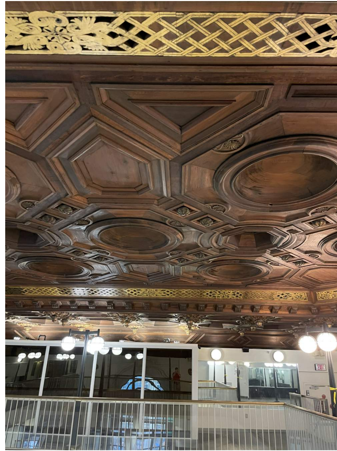
4 DECORATIVE CEILING FROM MEZZANINE 2 (2021)
