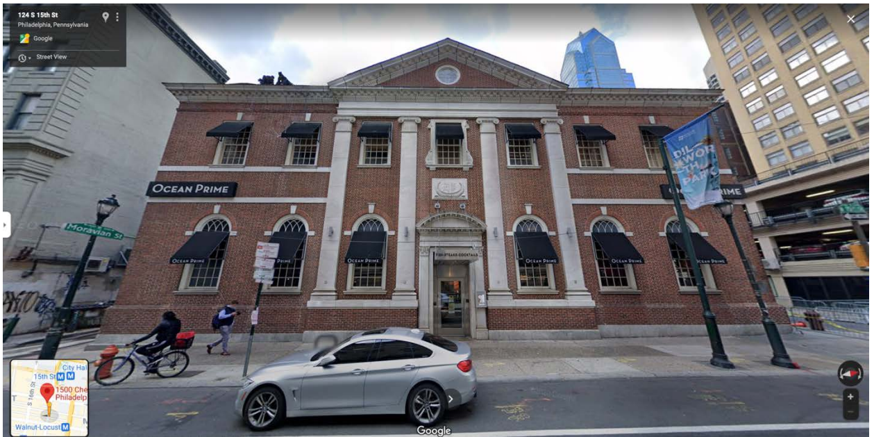
130 S. 15 TH STREET, NOVEMBER 2020: WINDOW OPENINGS CLOSED BACK UP
