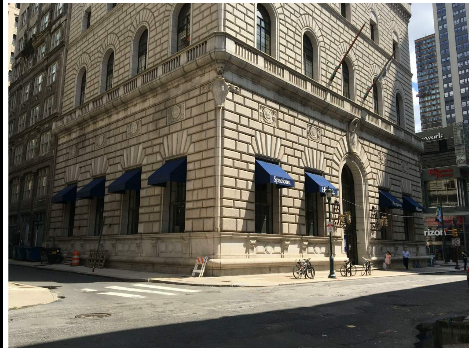
6 LOOKING SOUTHEAST FROM 15TH ST; MORAVIAN AT LEFT AND WALNUT AT RIGHT
