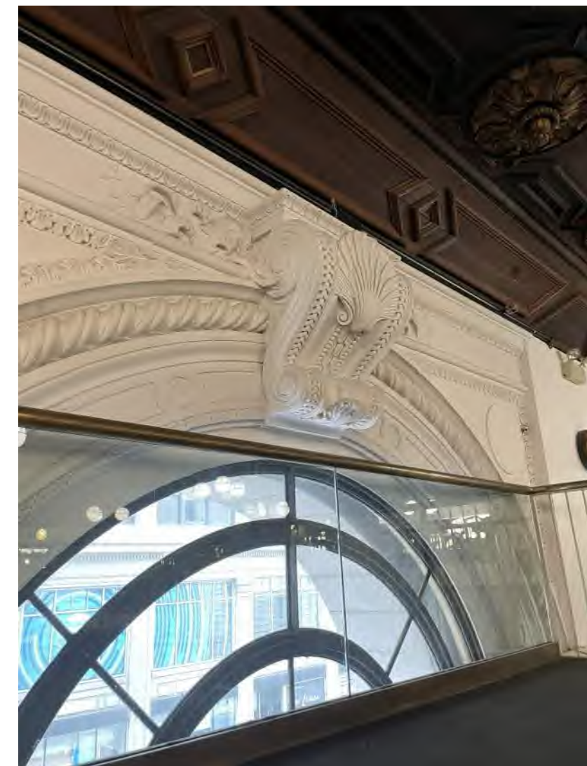
3 15TH ST ENTRY ARCH TOP VIEWED FROM MEZZANINE 2 (2021)
