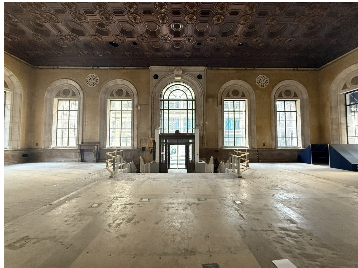
2 INTERIOR VIEW LOOKING WEST AT 15TH STREET ENTRY VESTIBULE (2025)
