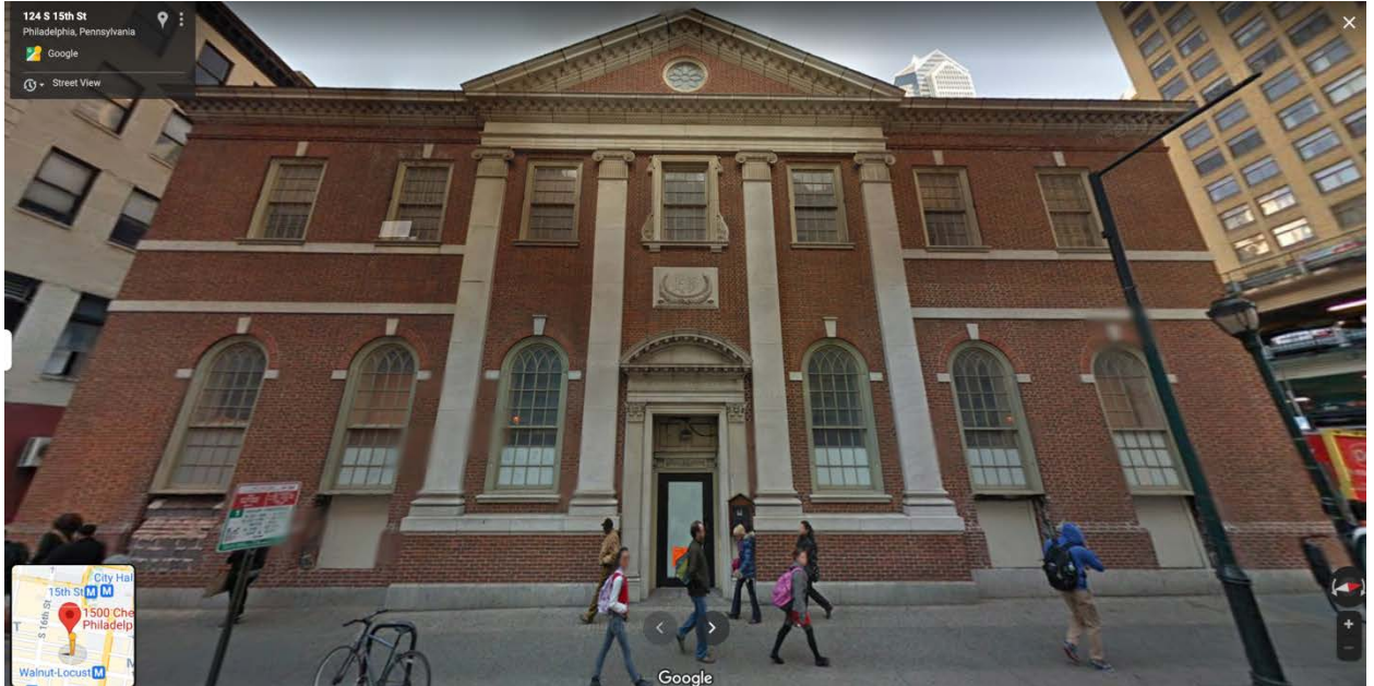
130 S. 15 TH STREET, MARCH 2012: LOWER LEVEL WINDOW OPENINGS UNDERGOING ENLARGEMENT
