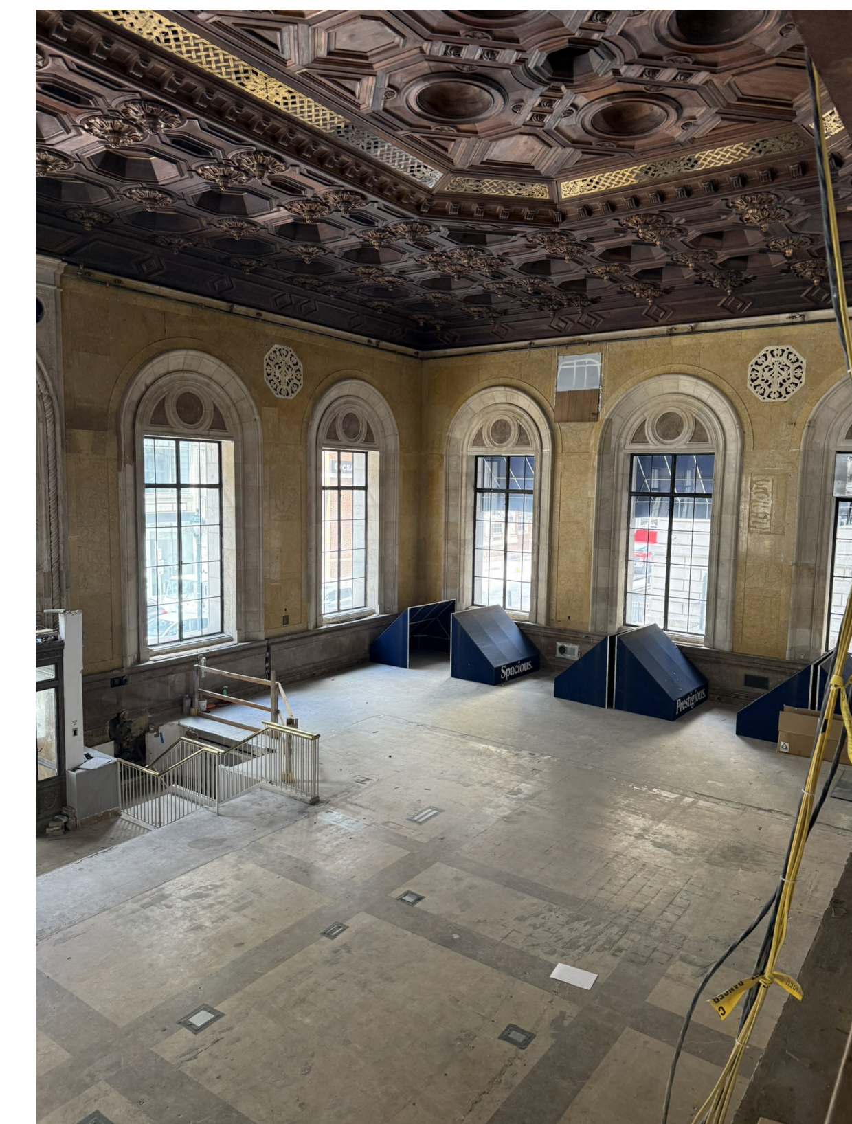
INTERIOR VIEW LOOKING NORTHWEST (2025)
