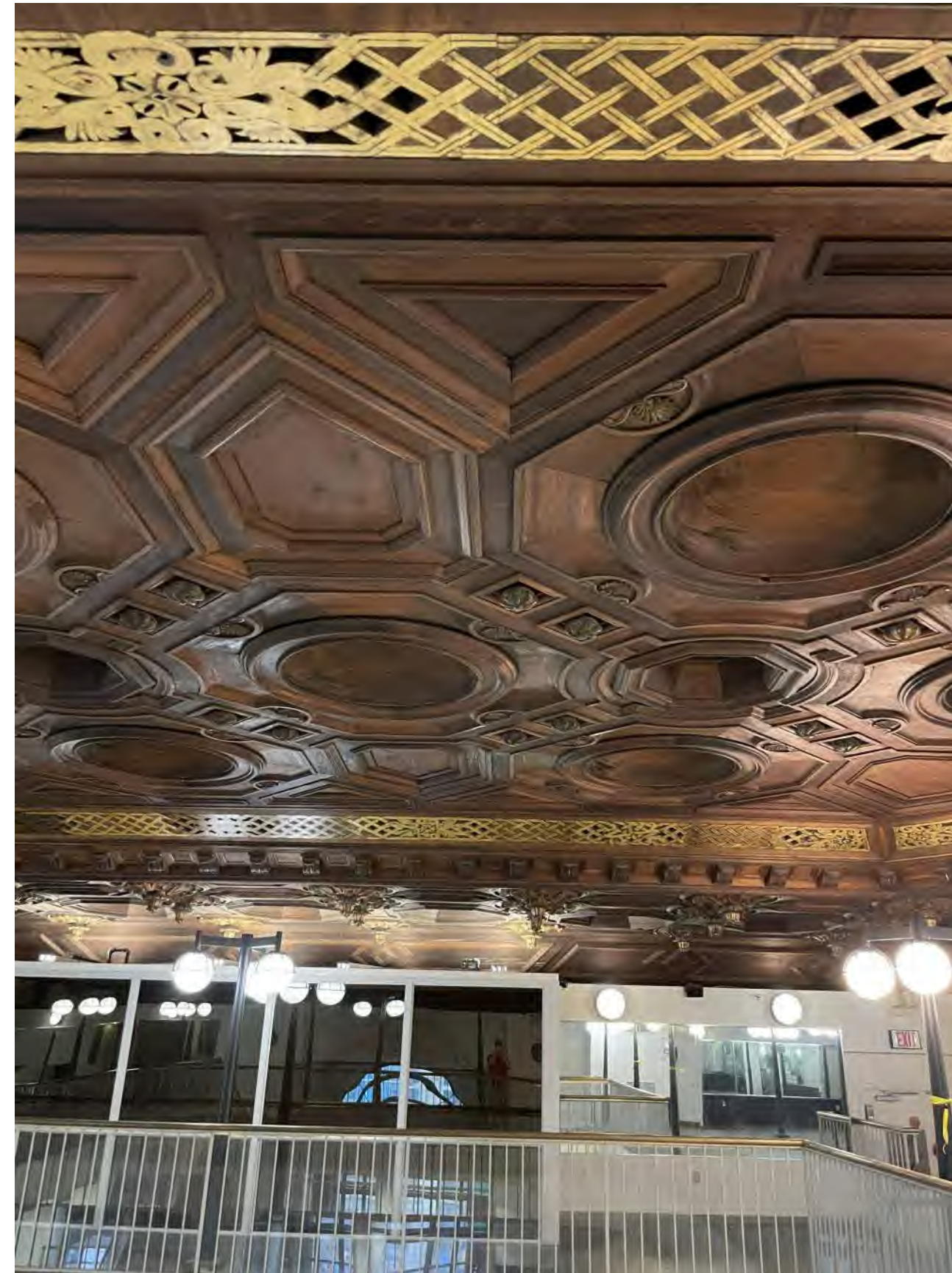
4 DECORATIVE CEILING FROM MEZZAINE 2 (2021)
