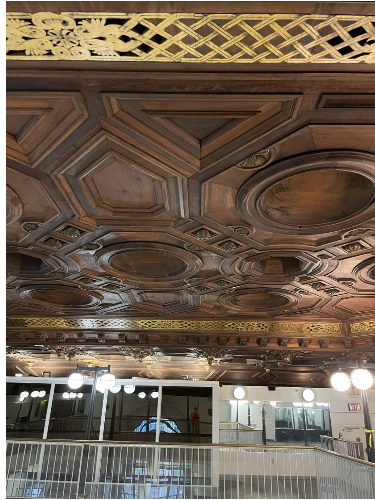
4 DECORATIVE CEILING FROM MEZZANINE 2 (2021)
