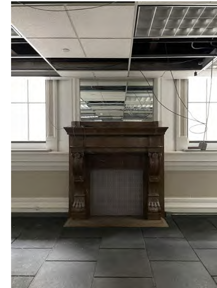
7 STONE FIREPLACE MANTEL (2021) (surrounding wall is original marble painted)
