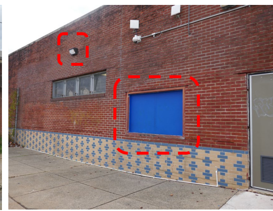
B. Existing surveillance opening & masonry damage, building-mounted exterior lights
