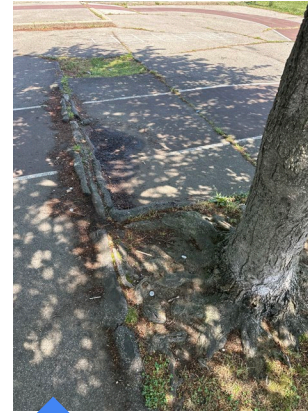
Tree 3; roots heaving asphalt
