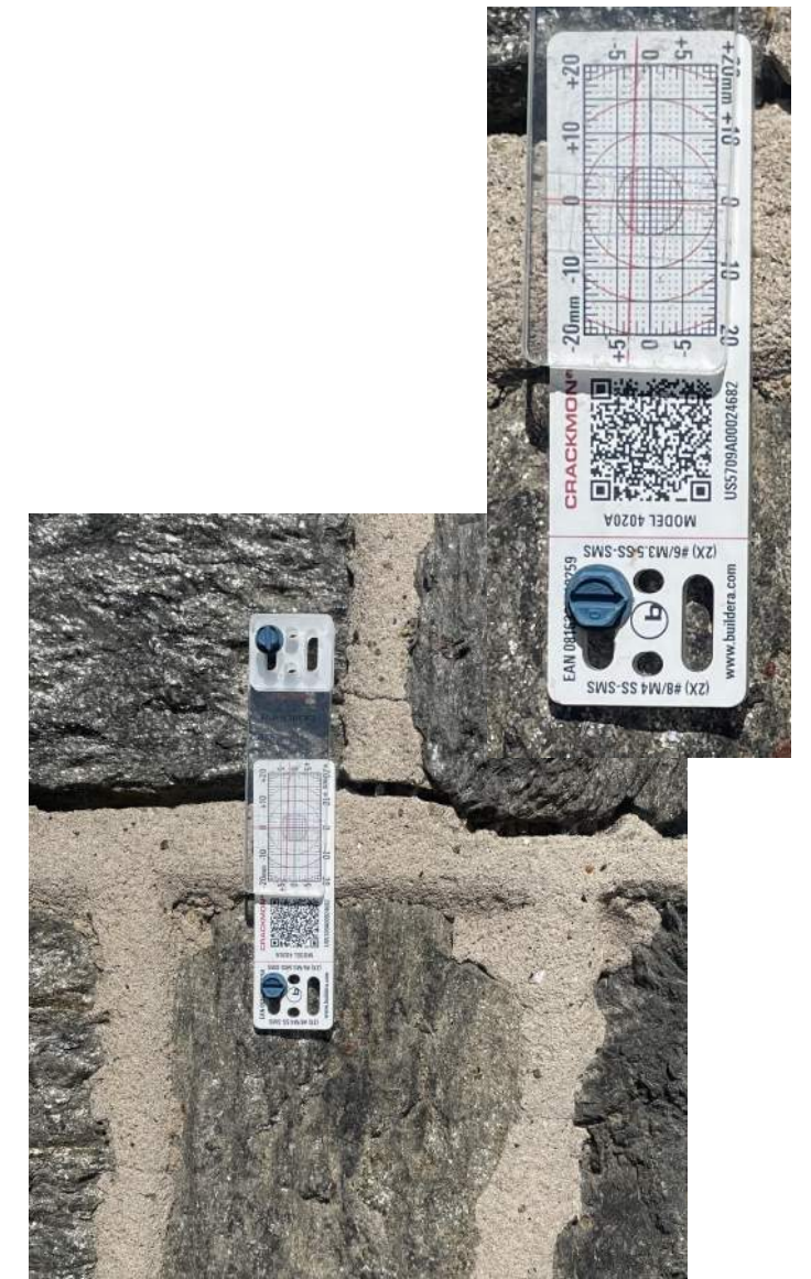
GAUGE AT UPRIVER PIER 23 FEB 2025
