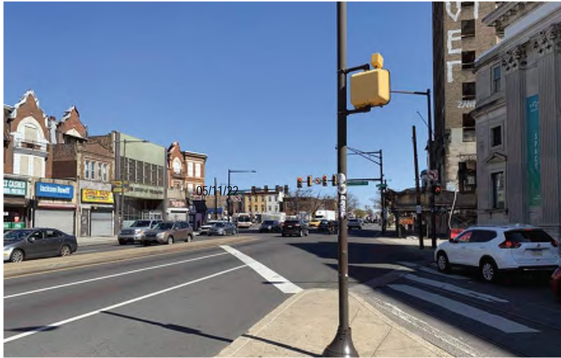
VIEW FROM ISLAND LOOKING NORTH
