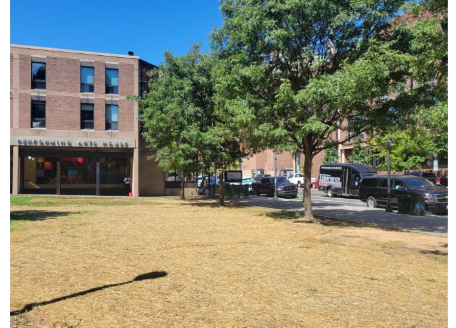
VIEW FROM EAST GRASS COURTYARD LOOKING WEST AT WB-1 STAIRCASE AND SPRUCE ST
