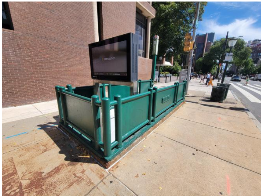
VIEW FROM WEST SPRUCE ST LOOKING AT WB-2 STAIRCASE
