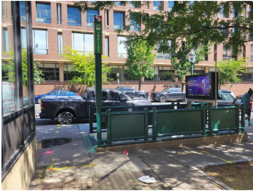
VIEW FROM WEST GRASS COURTYARD LOOKING NORTH AT WB-1 STAIRCASE
