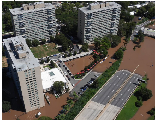
Schuylkill River flooding
