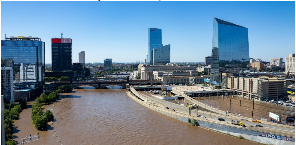
Figure 18: Interstate 676 after Hurricane Ida
