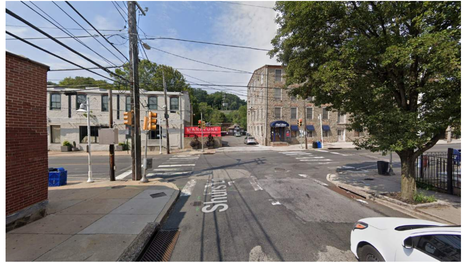
2 View of Site from Shurs Lane looking South
