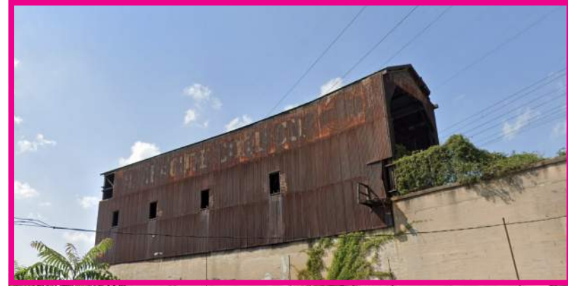
Corrugated Metal Siding at Nearby Rail Spur
