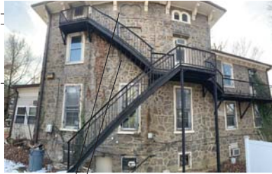
WINDOW SHAPED STONE RECESSES EXIST ON RIGHT SIDE FACADE OF BUILDING, BUT NOT ON LEFT SIDE FACADE OF BUILDING
