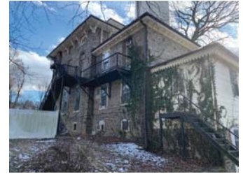
WINDOW SHAPED STONE RECESSES EXIST ON RIGHT SIDE FACADE OF BUILDING, BUT NOT ON LEFT SIDE FACADE OF BUILDING
