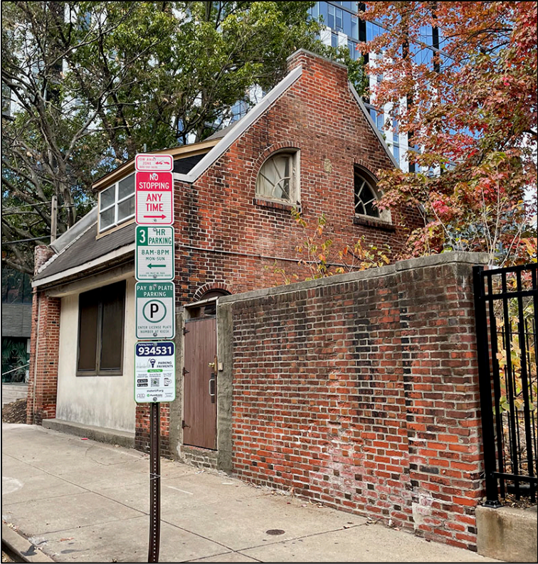
Fig. 11. Rear garage along Sansom Street showing east (gable end) and south elevations. The gate to the east of the garage opens to a brick path toward the main building. Date: November 1, 2024.
