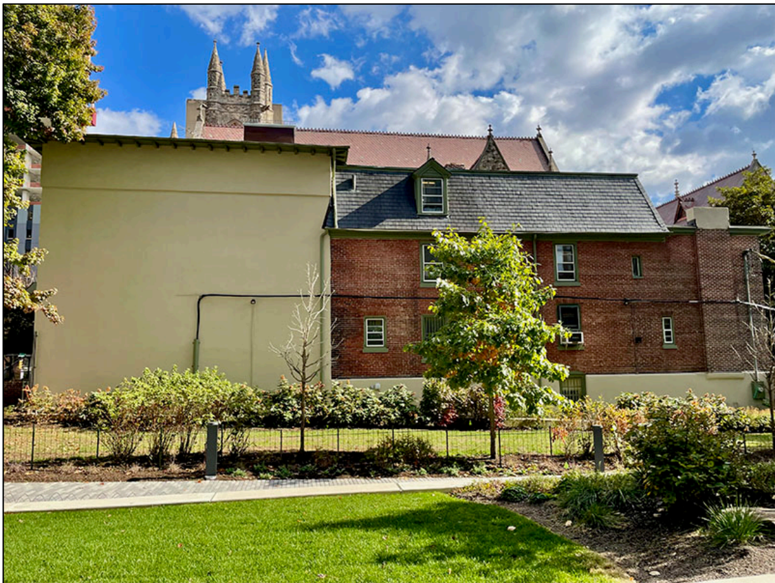
Fig. 6. West elevation showing main volume (left) and later additions. Date: November 1, 2024.
