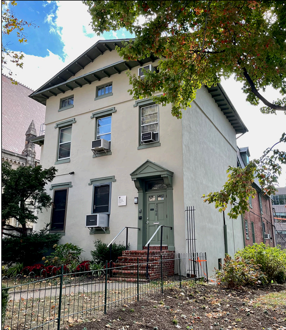
Fig. 4. Primary elevation of the subject property. Date: November 1, 2024.
