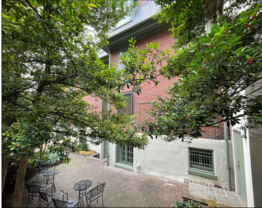
Fig. 8. East elevation of the additions to the south of the original villa facing the rear courtyard. Date: December 17, 2023.
