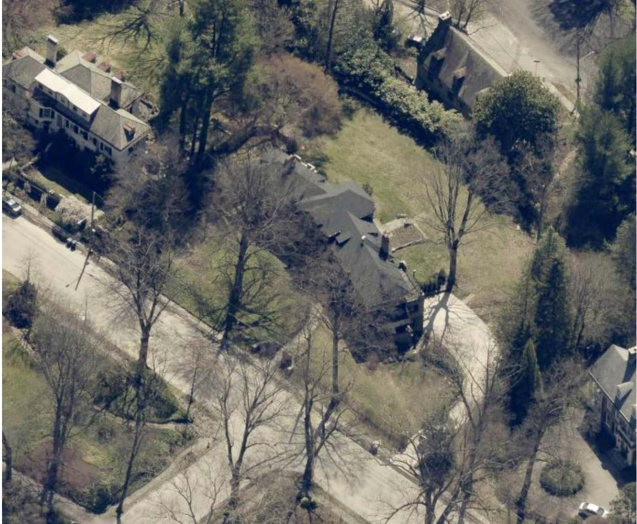
Figure 3. Aerial view of 7716 Navajo Street, looking south. Source: Pictometry.
