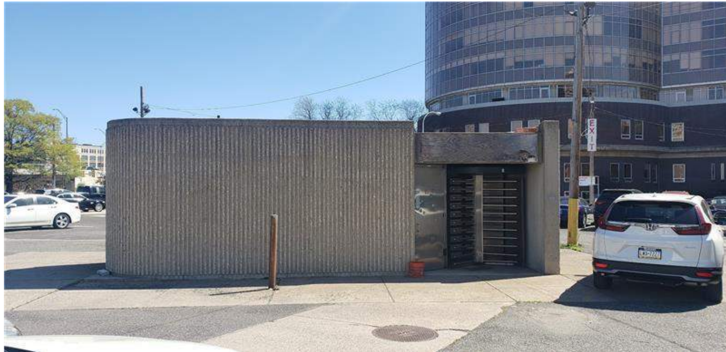
VIEW OF EAST EXISTING EGRESS STAIR HEADHOUSE LOOKING NORTHEAST
