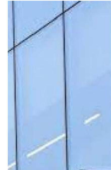
CLERESTORY GLASS STOREFRONT
