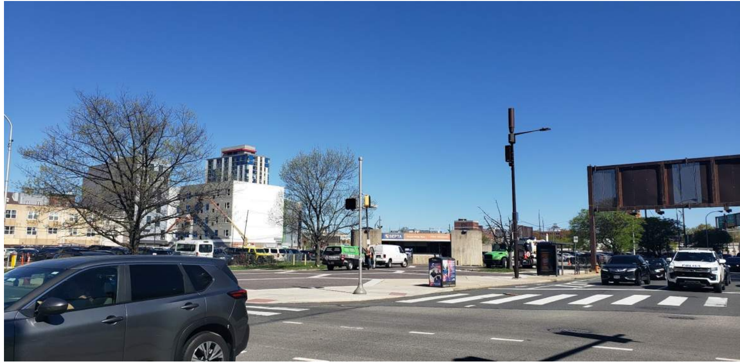
VIEW OF HEADHOUSE LOOKING NORTHWEST FROM THE INTERSECTION OF RACE & N 8TH STREETS
