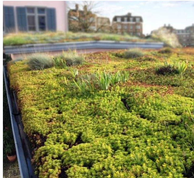
GREEN ROOF EXTENSIVE
