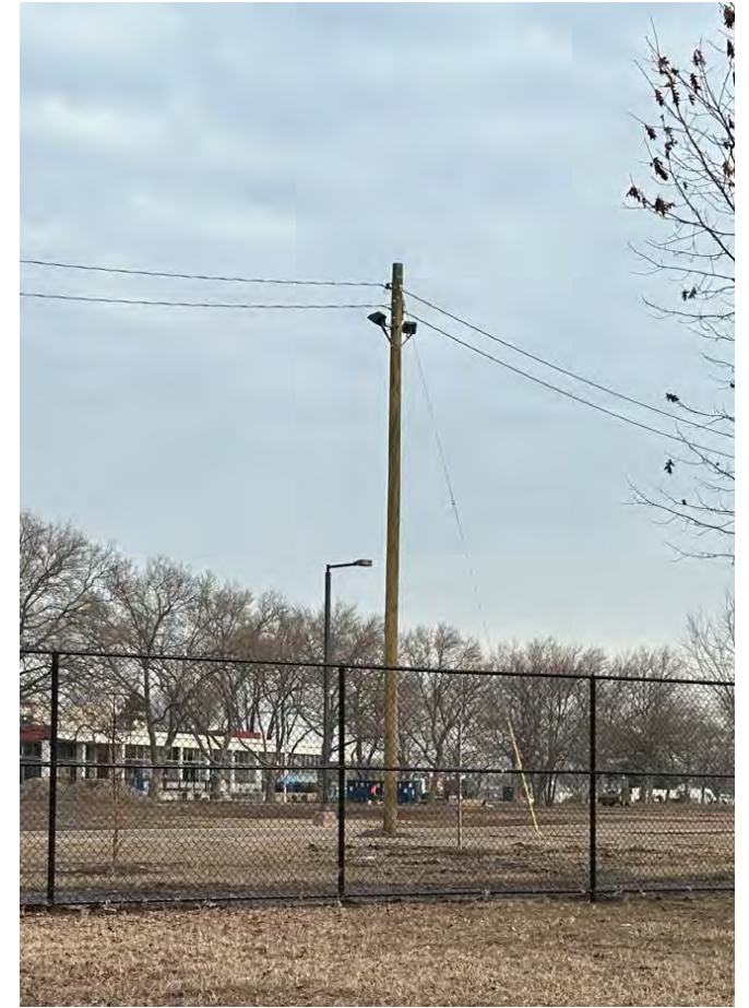
Security Fence and Lighting
