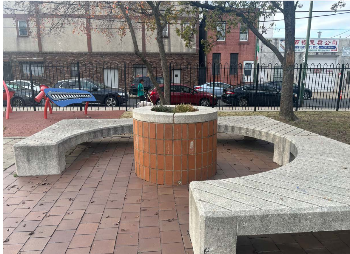
Existing benches and planters to be removed
