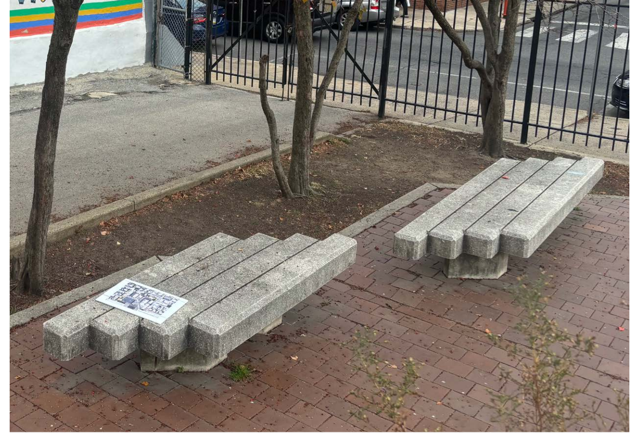
Existing benches to be removed
