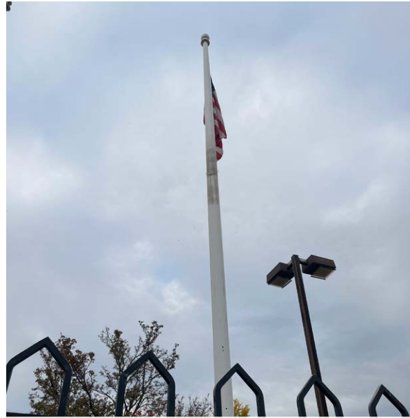
Existing flagpole to be relocated; existing lightpole to be replaced
