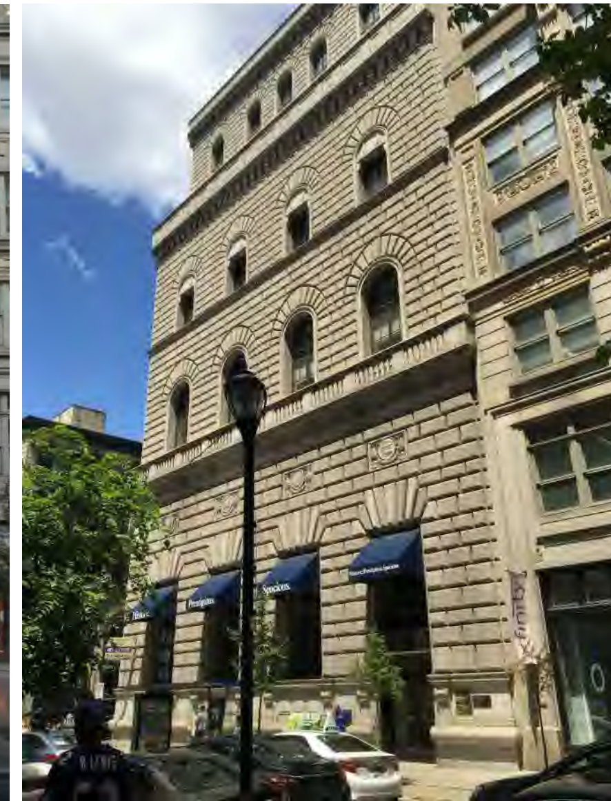
5 LOOKING NORTHWEST AT WALNUT STREET FACADE
