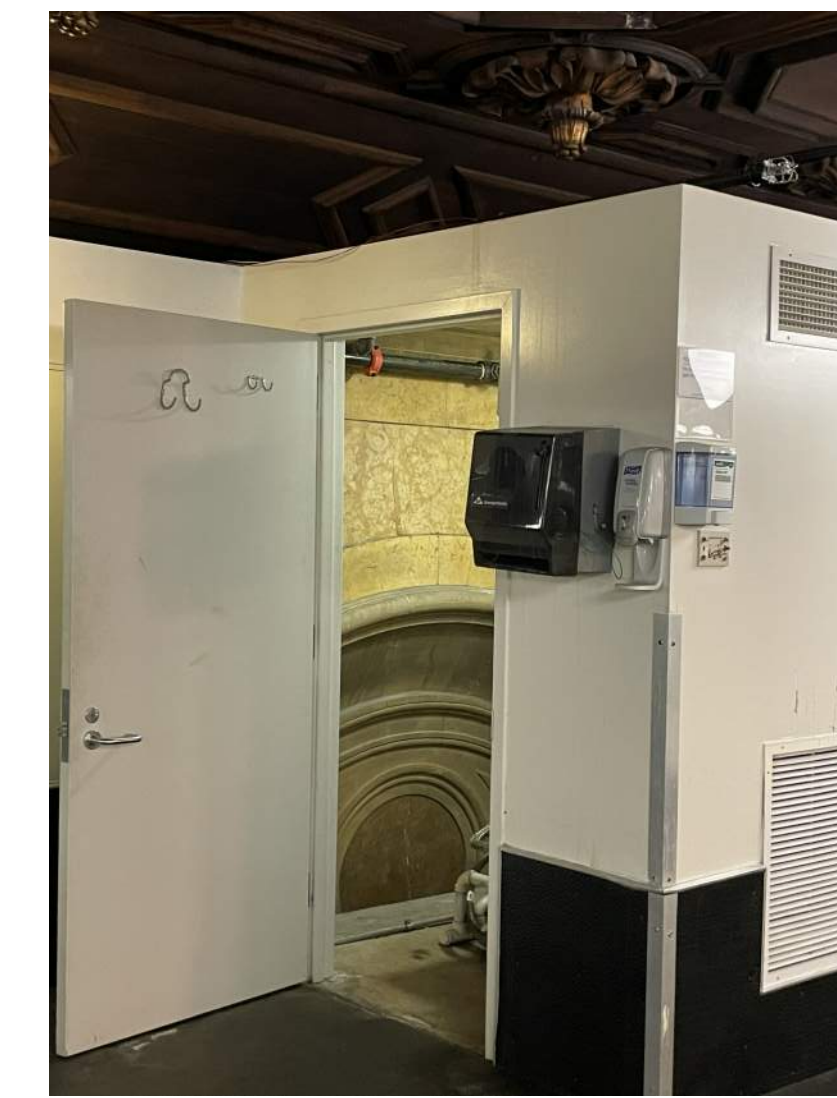
8 STONE ROUND TOP OF TYP. WINDOW VIEWED ON MEZZANINE 2 (2021)
