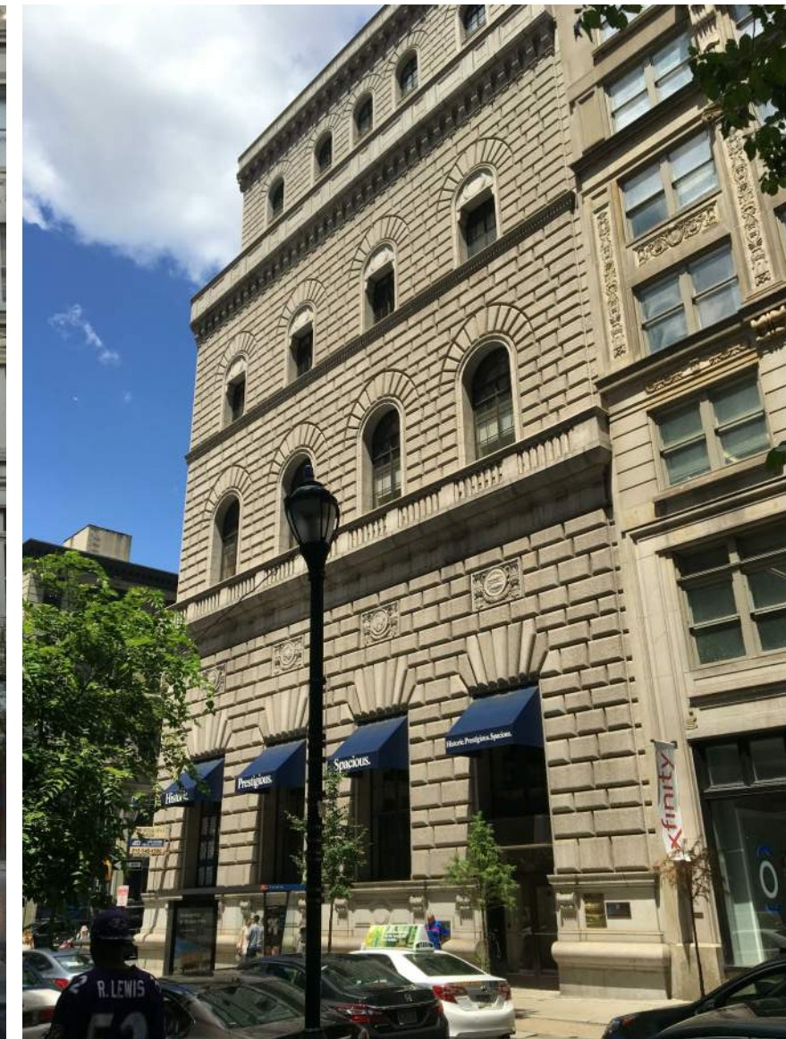
5 LOOKING NORTHWEST AT WALNUT STREET FACADE
