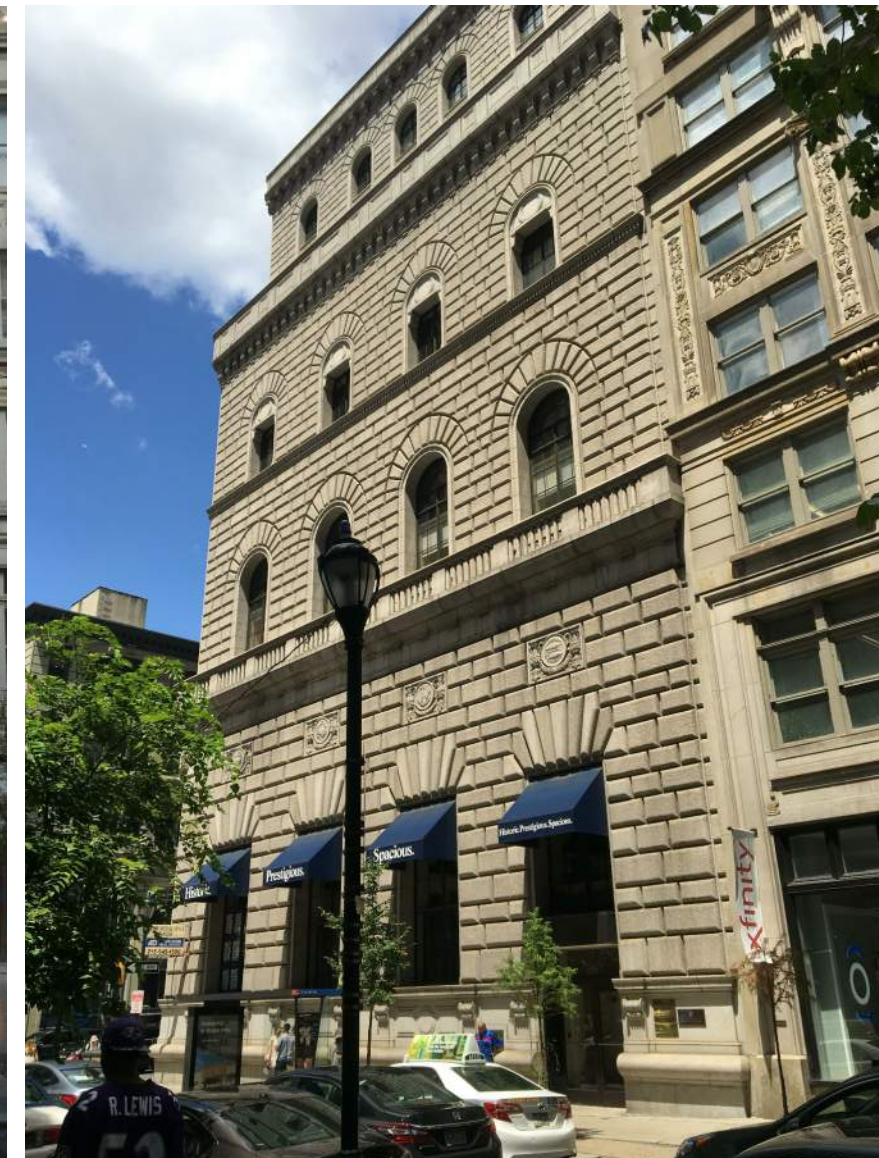
5 LOOKING NORTHWEST AT WALNUT STREET FACADE
