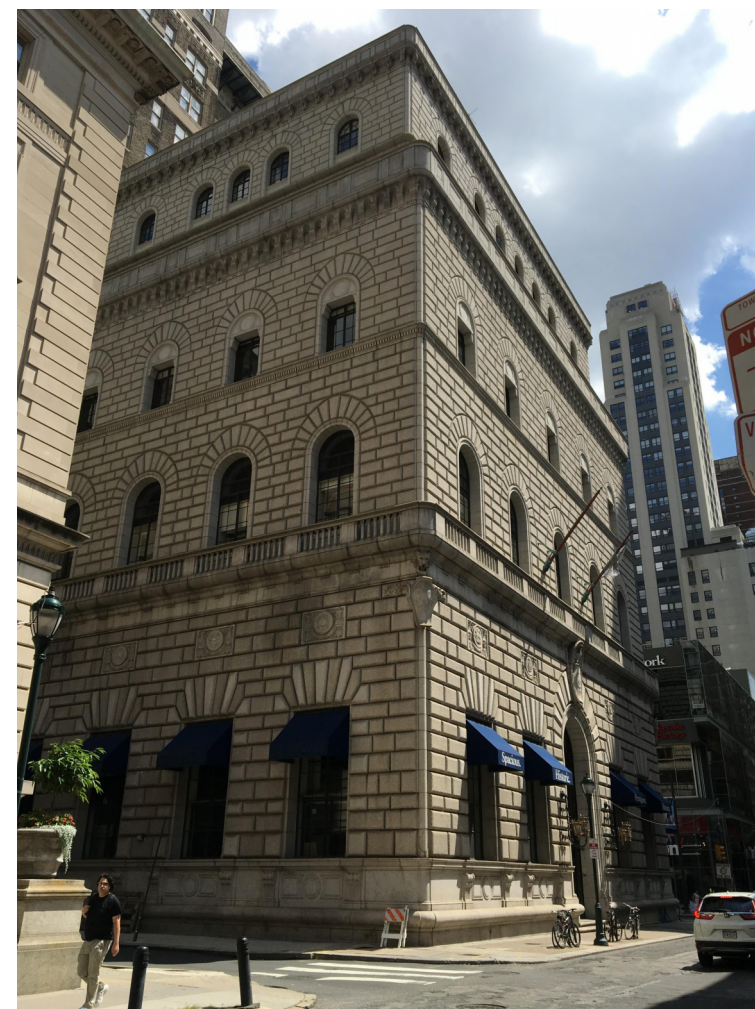
LOOKING SOUTH TO CORNER OF 15TH AND MORAVIAN
