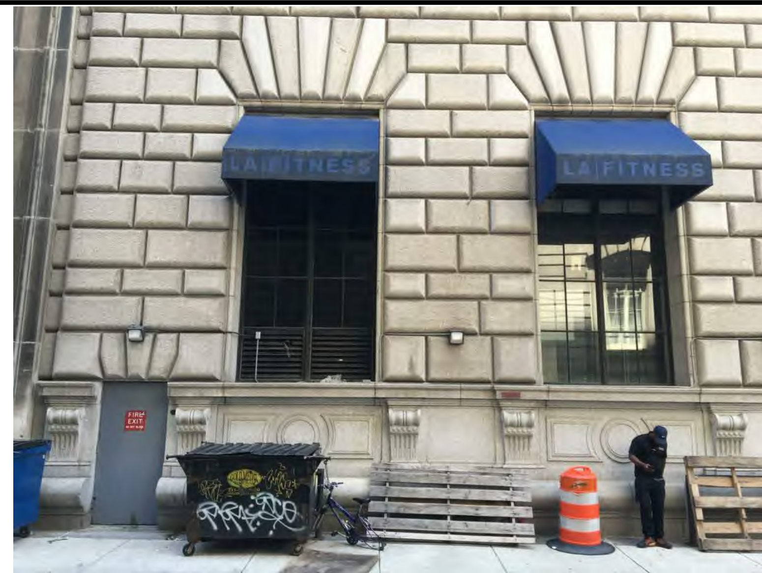
11 MORAVIAN STREET PARTIAL FACADE - FIRE EGRESS AT LEFT
