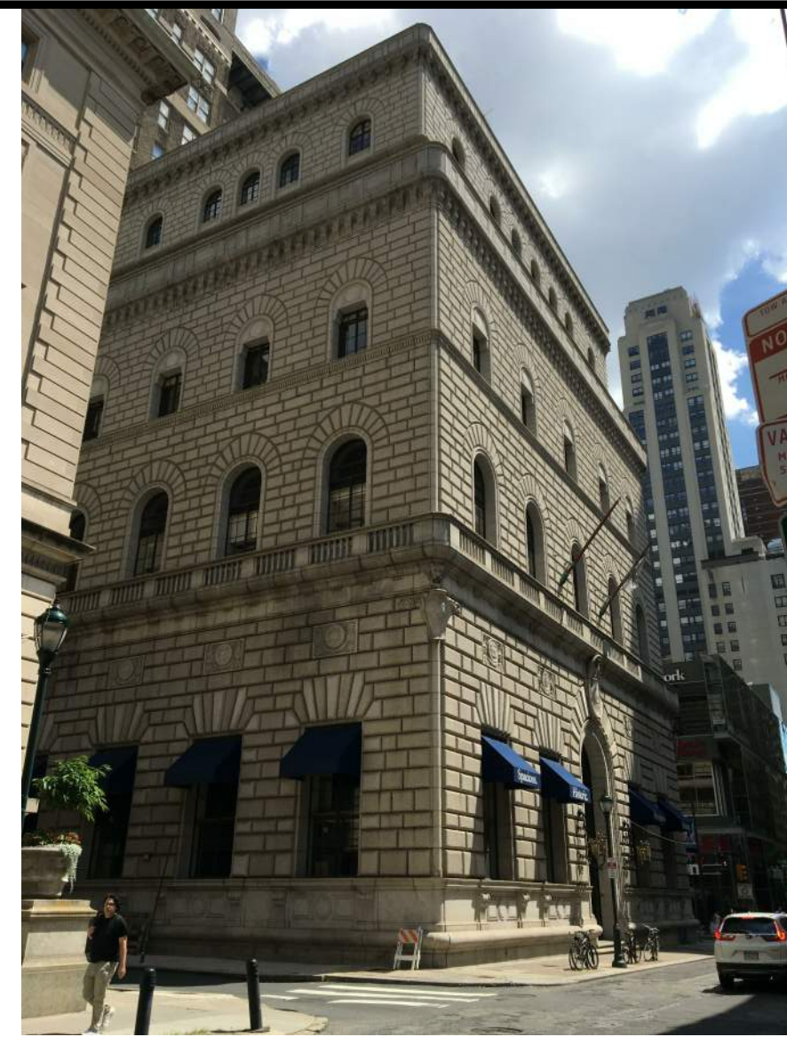
10 LOOKING SOUTH TO CORNER OF 15TH AND MORAVIAN
