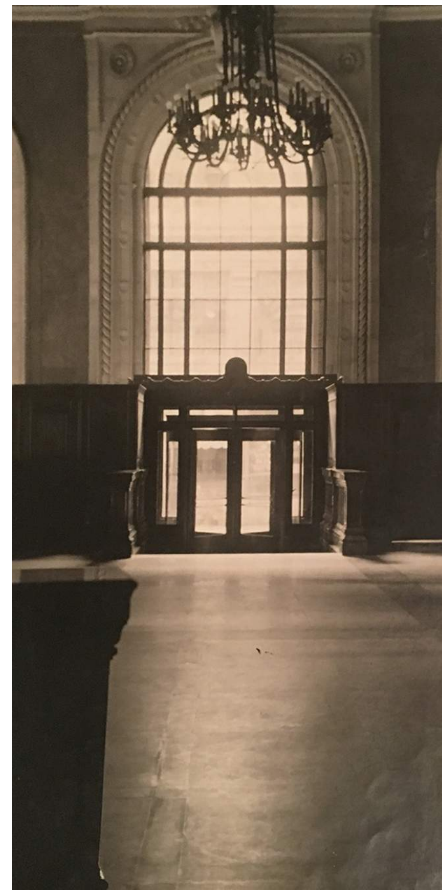
2 15TH STREET ENTRANCE INTERIOR VIEW CIRCA 1928
