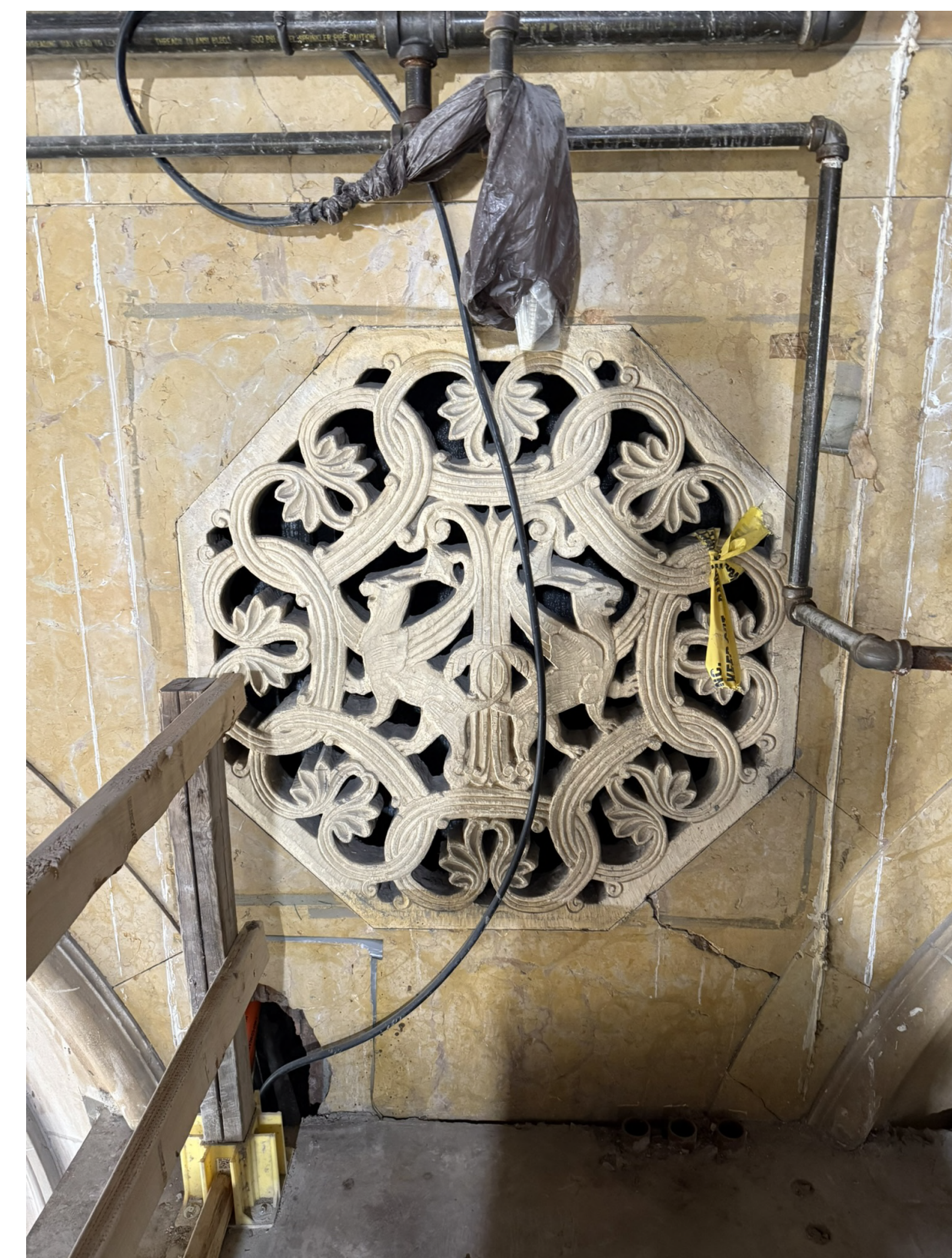
VENT DETAIL BETWEEN WINDOW ARCHES (2025)
