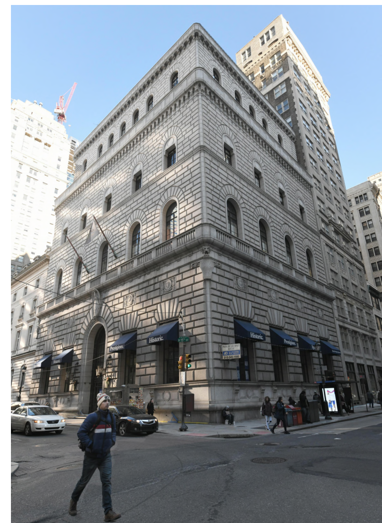
LOOKING AT NORTHEAST CORNER OF 15TH AND WALNUT
