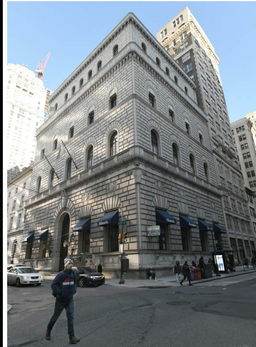
1 LOOKING AT NORTHEAST CORNER OF 15TH AND WALNUT
