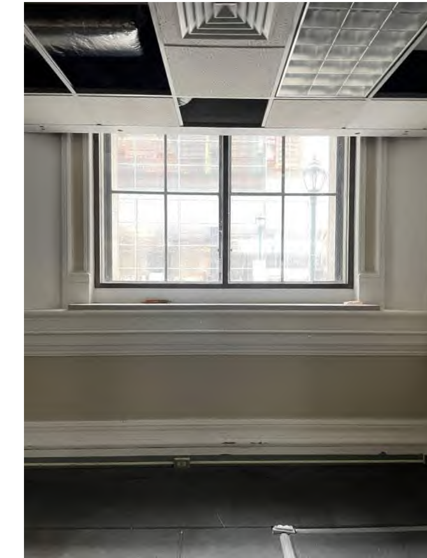
10 LOWER PORTION OF TYPICAL WINDOW AT FIRST FLOOR (2021)
