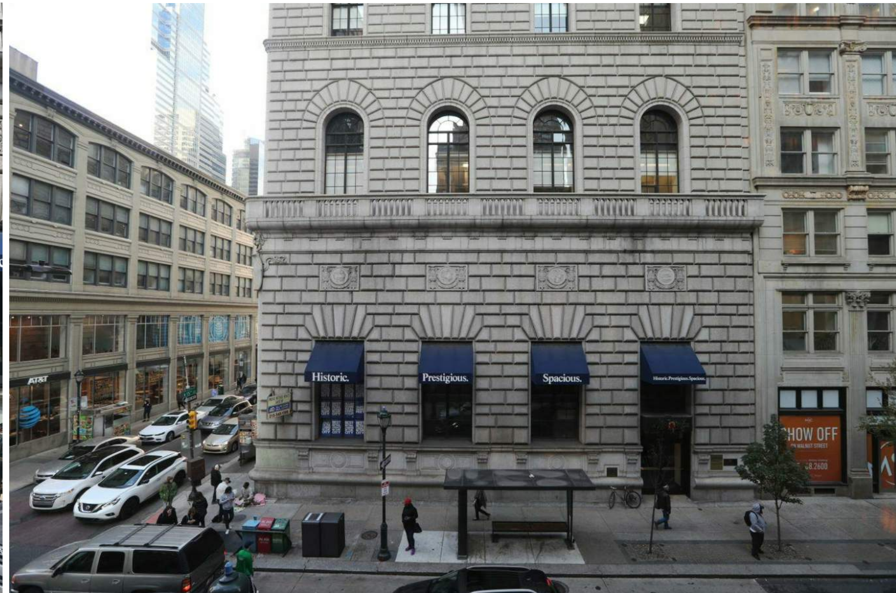
4 WALNUT STREET FACADE
