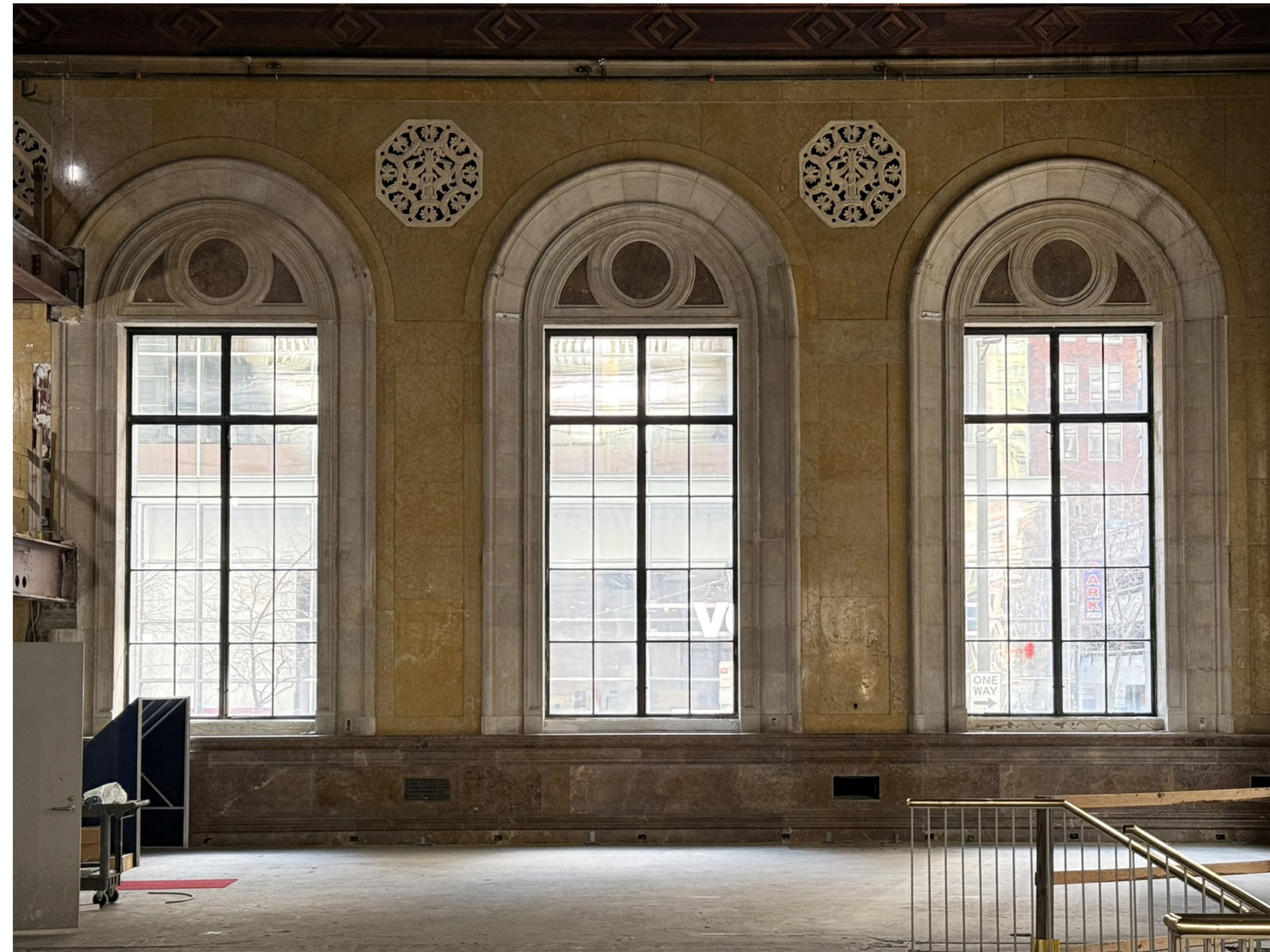
WALNUT STREET WINDOWS FROM INTERIOR (2025)
