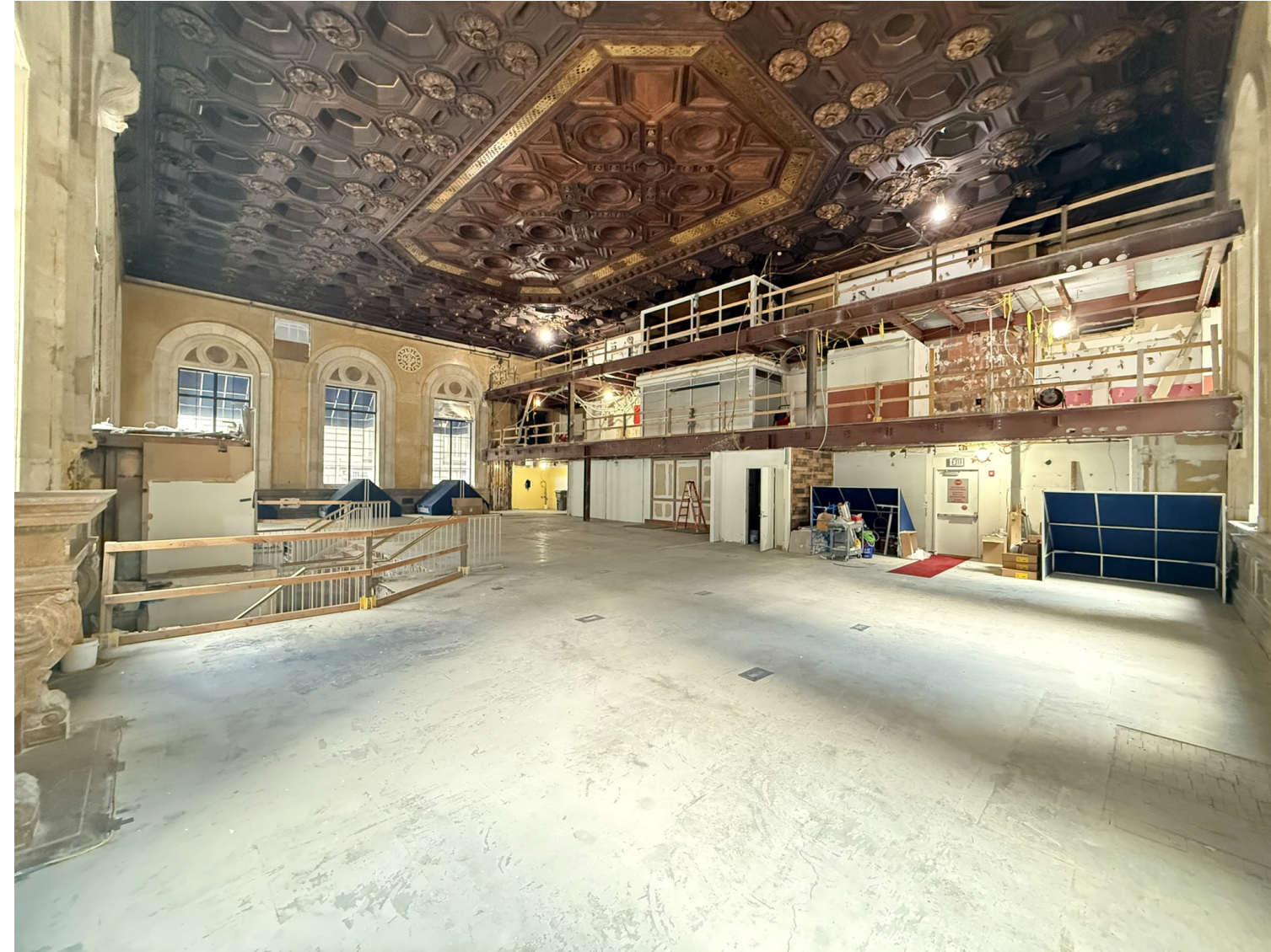
1 INTERIOR VIEW LOOKING NORTHEAST (2025)
