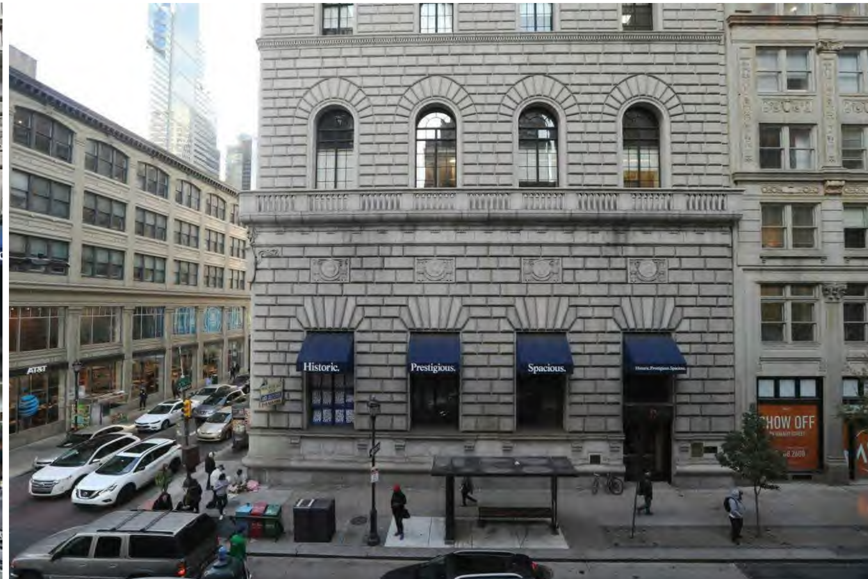
4 WALNUT STREET FACADE
