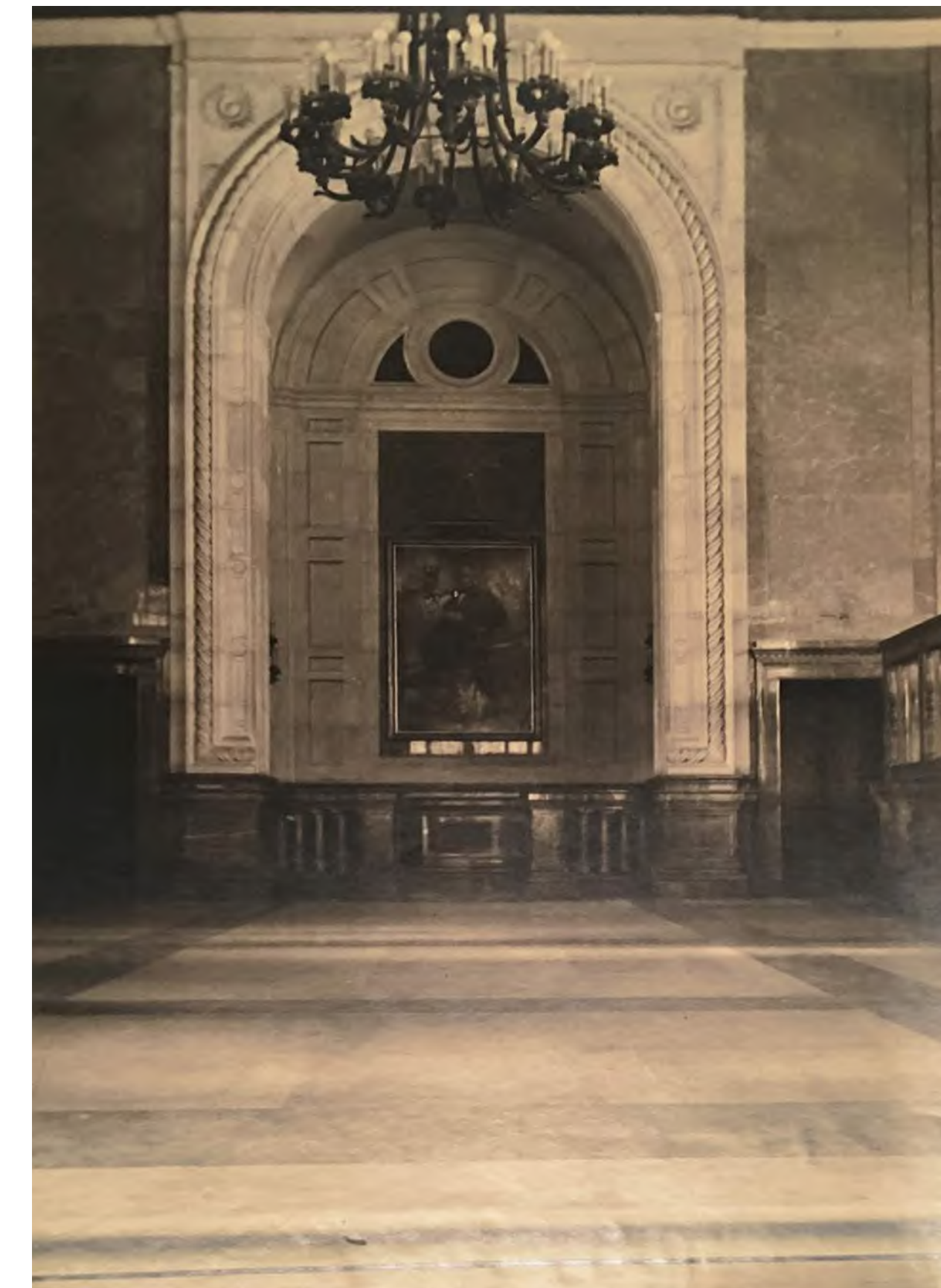
6 CENTER NICHE VIEWED FROM 15TH STREET ENTRANCE CIRCA 1928
