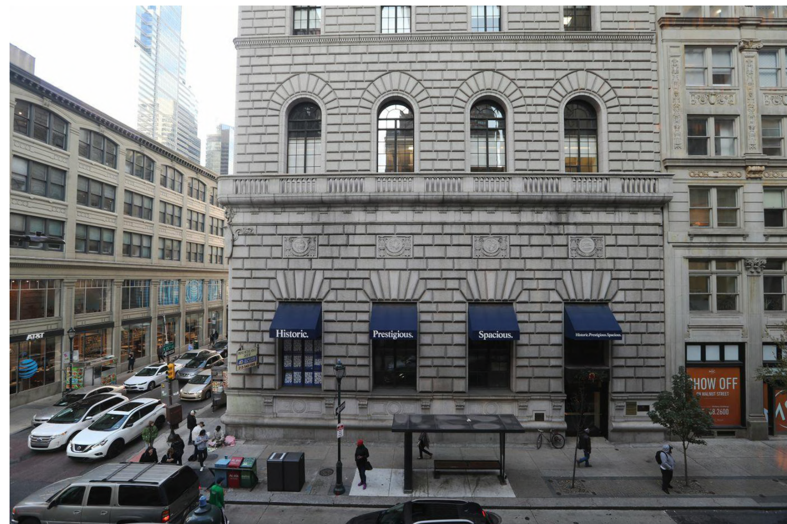
WALNUT STREET FACADE
