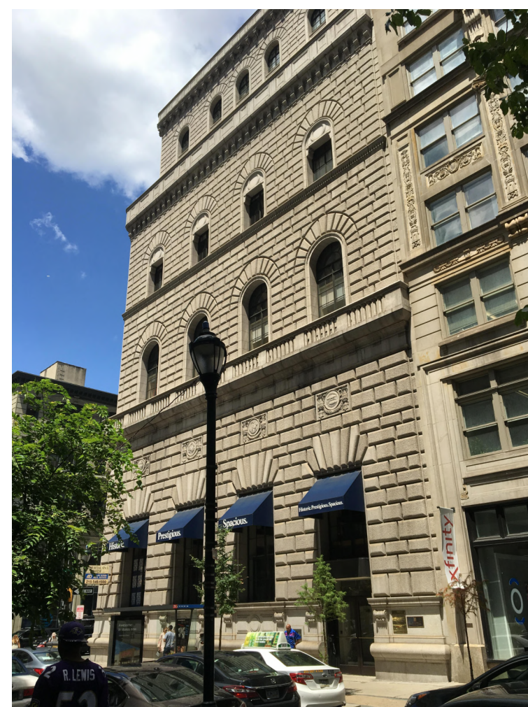
LOOKING NORTHWEST AT WALNUT STREET FACADE
