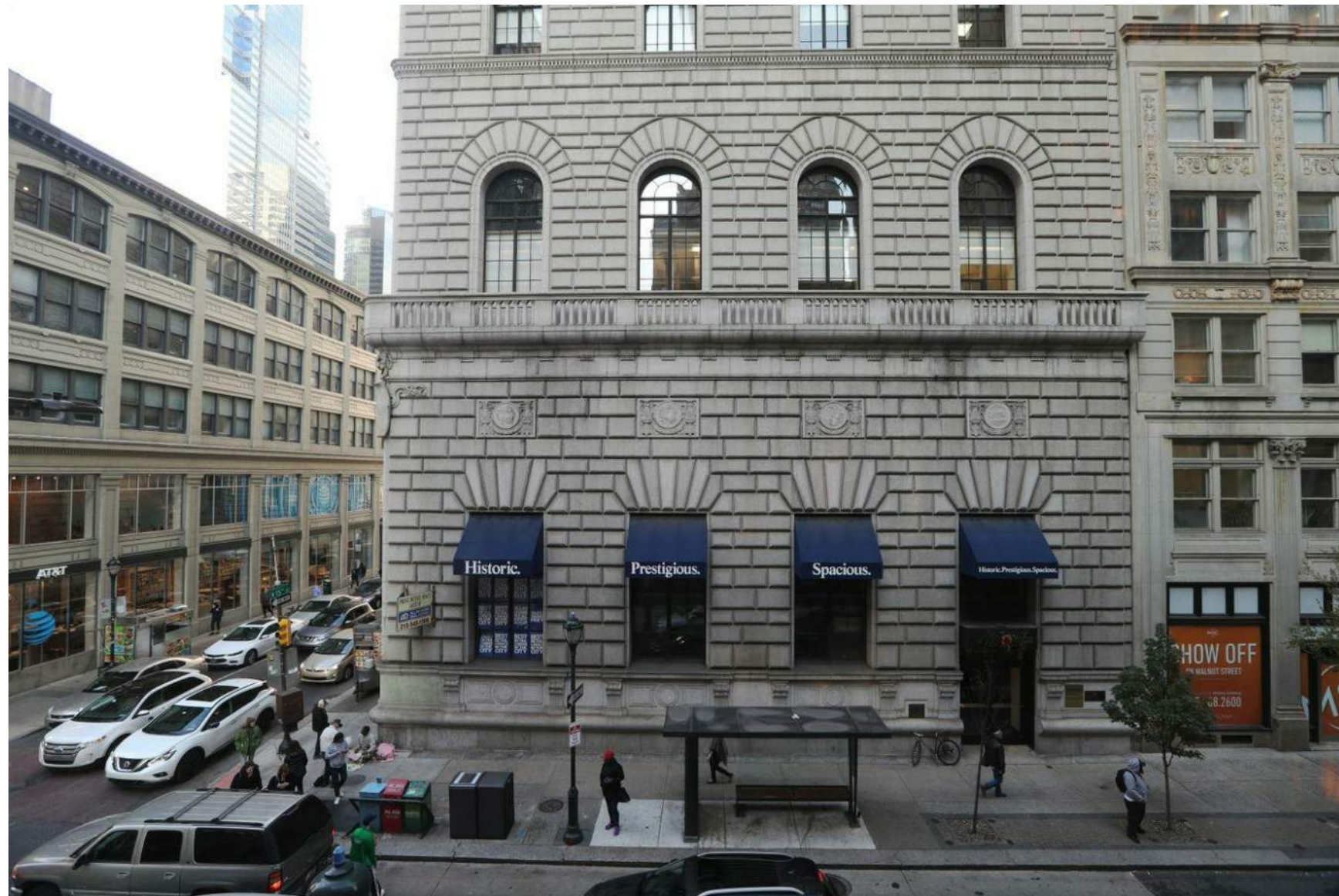
4 WALNUT STREET FACADE
