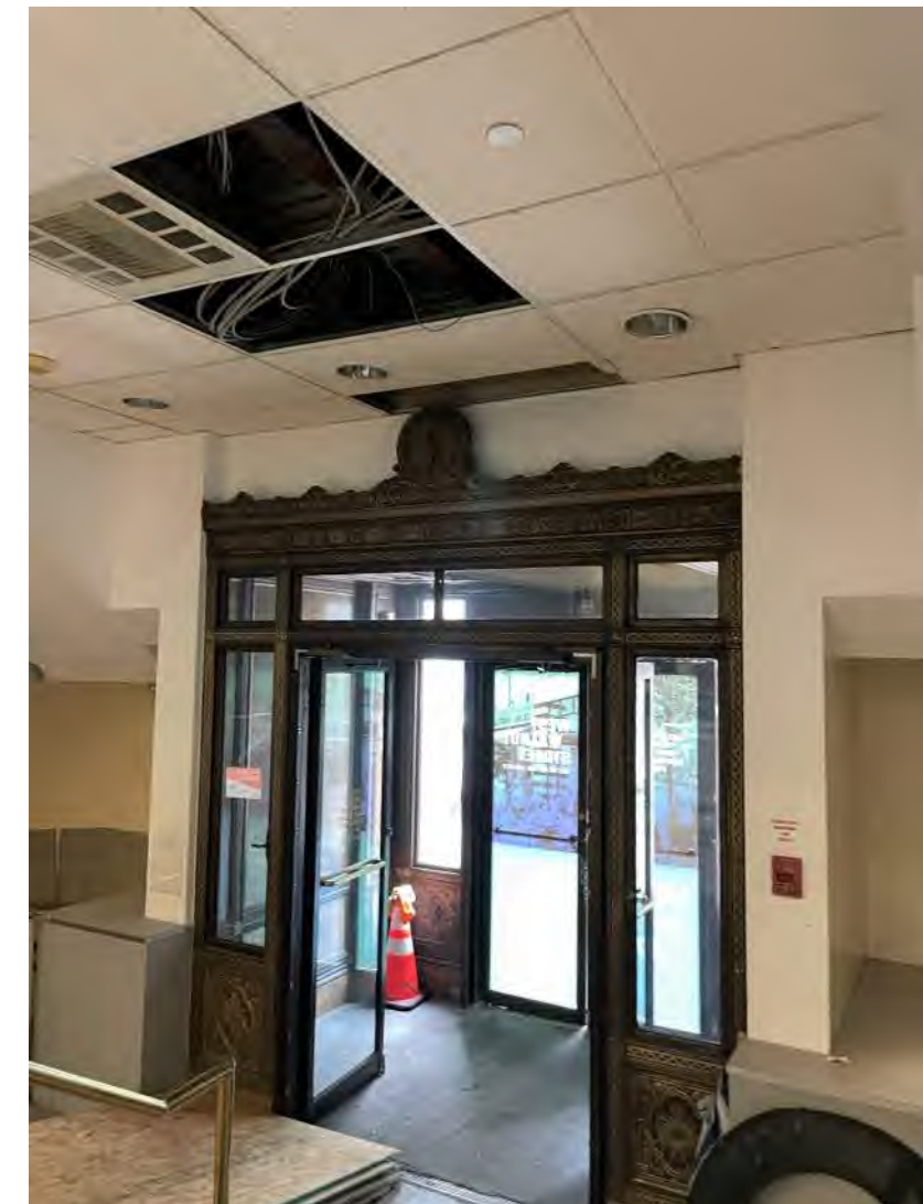
4 DECORATIVE METAL VESTIBULE FROM FIRST FLOOR (2021)
