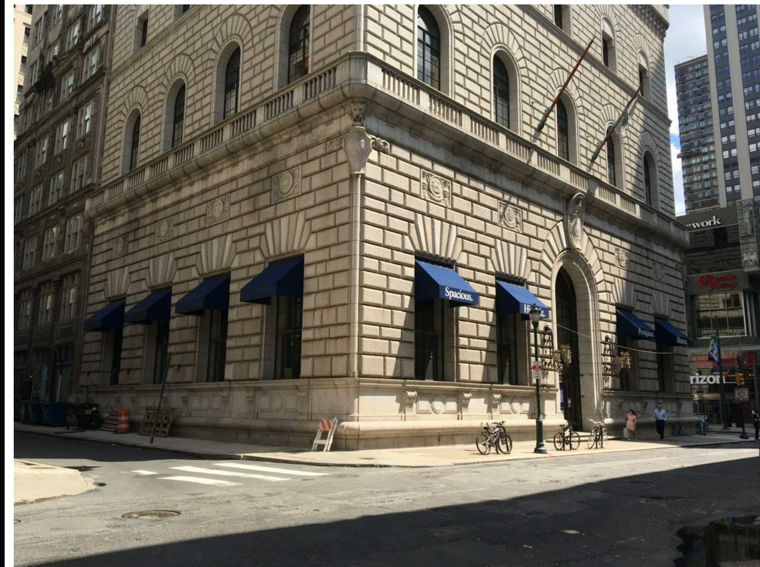
6 LOOKING SOUTHEAST FROM 15TH ST; MORAVIAN AT LEFT AND WALNUT AT RIGHT
