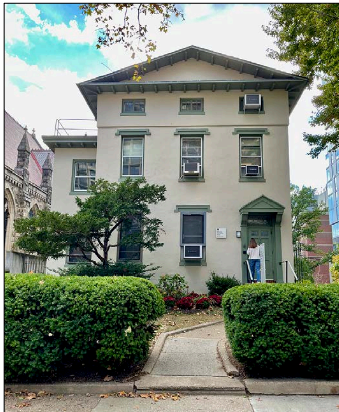
Fig. 5. Primary elevation along Chestnut Street. Date: November 1, 2024.
