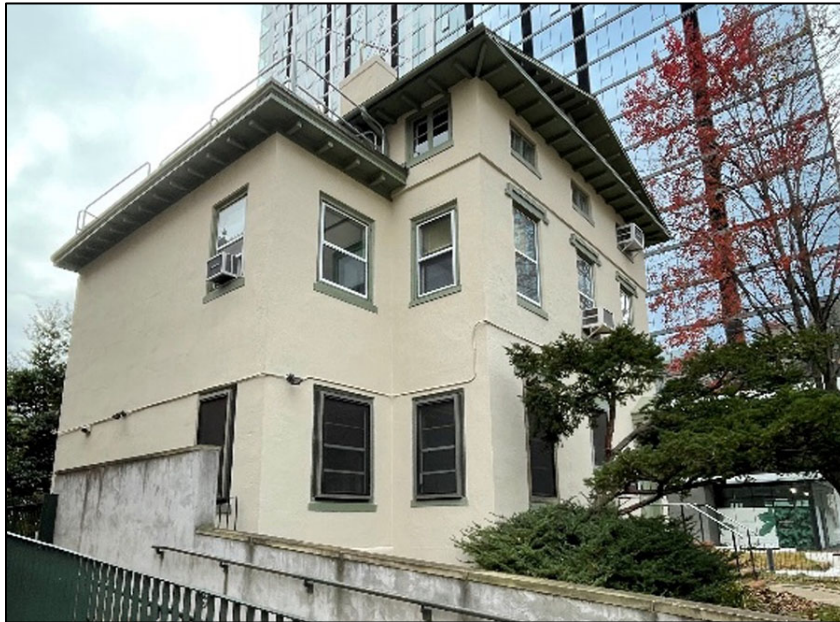
Fig. 9. East elevation of the original villa from the ramp of the church to the east. Date: December 17, 2023.
