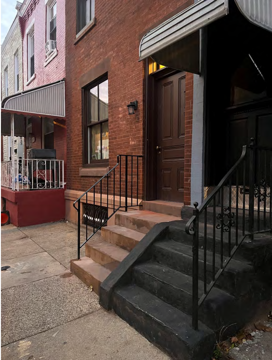
40 - Railing Addition (photo by Massoud Mohadjeri), November 2025
