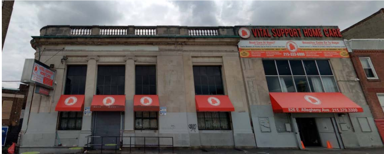
Figure 2. 820-26 E. Allegheny Ave. August 2024. Source: Cyclomedia
