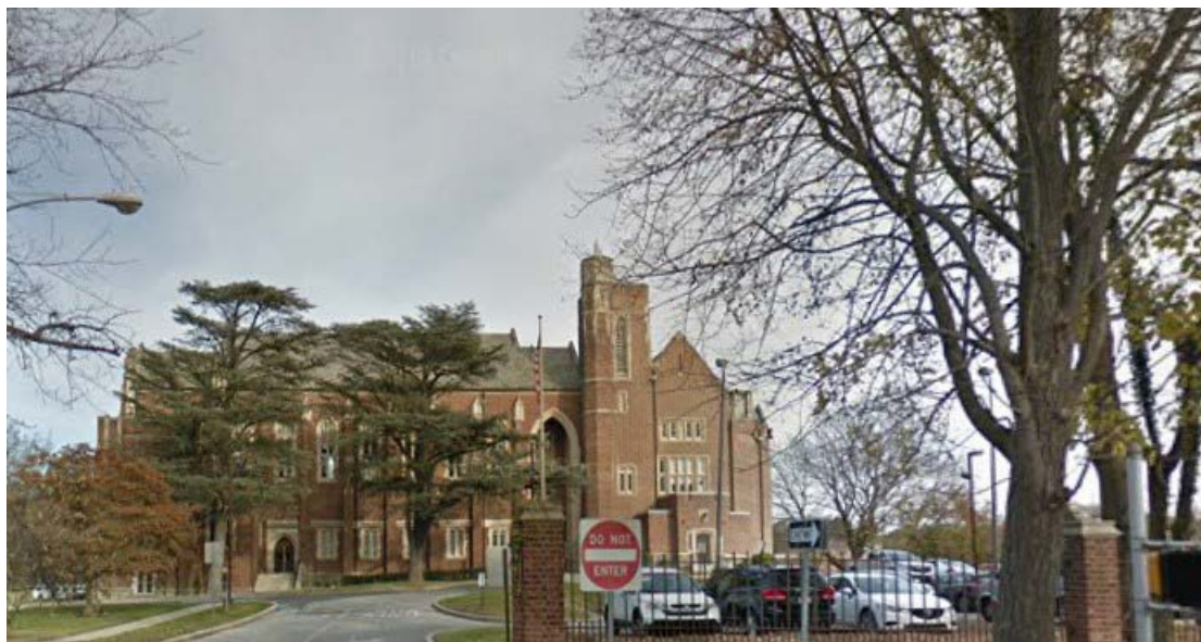
Figure 53. Academy of Sacred Heart (Perelman Jewish Day School), Overbrook, PA. Paul Monaghan, Architect, 1923. Source: Google Streetview
