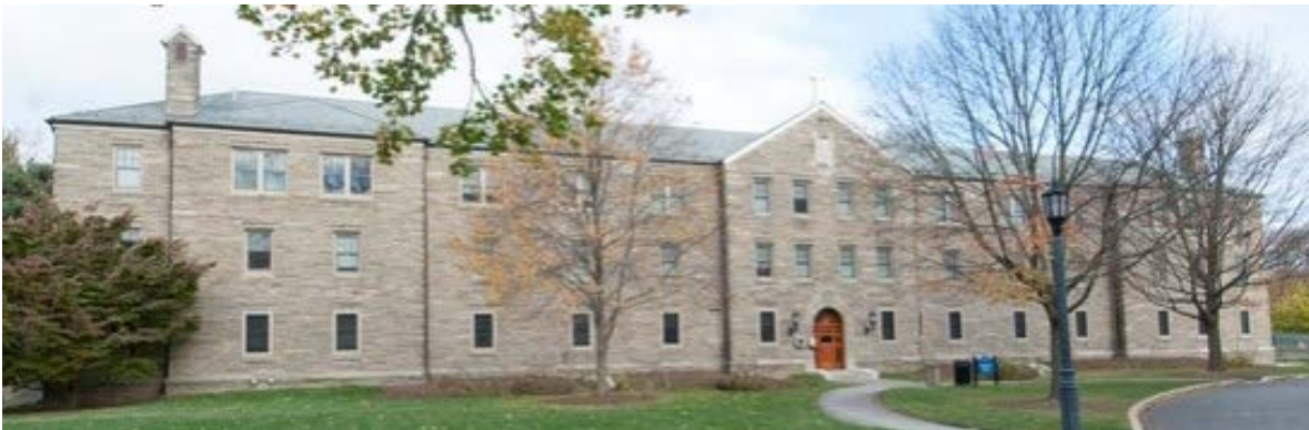
Figure 67. Ferdigan Hall Dormitory, Villanova, PA. Paul Monaghan, Architect, 1928. Source: villanov.edu.
