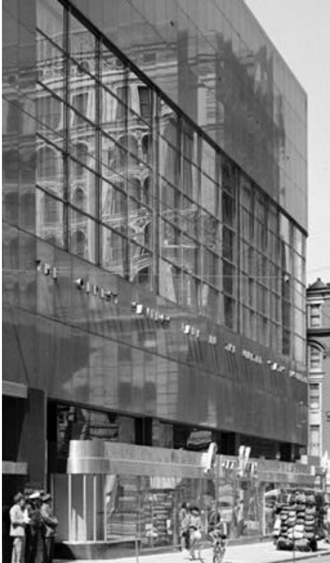
Figure 24. Detail of S. 12th Street Glazing, PSFS Building, 1200 Market Street. Howe and Lescaze – 1932. Source: adaptandreuse.com/philadelphia-pdfs-building-is-now-a-loews-hotel .
