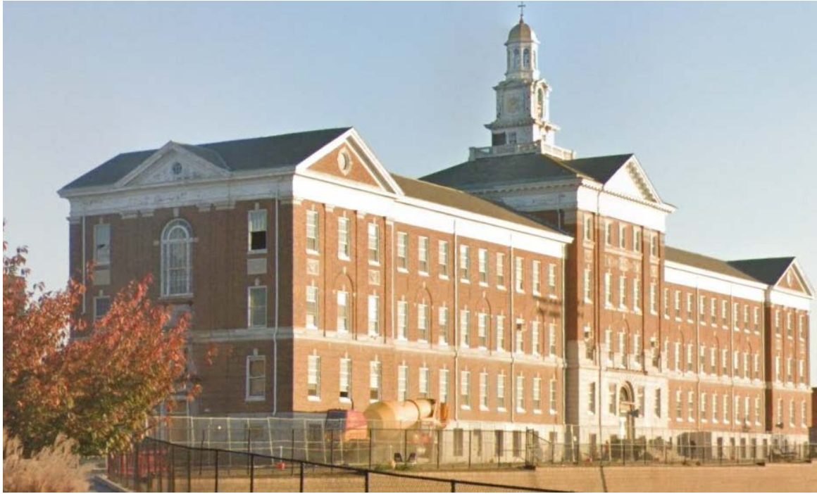
Figure 61. St. Vincent Home, Now Msgr. Bonner and Abp. Pendergast HS, Paul Monaghan, Architect 1920. Source: Google Streetview.
