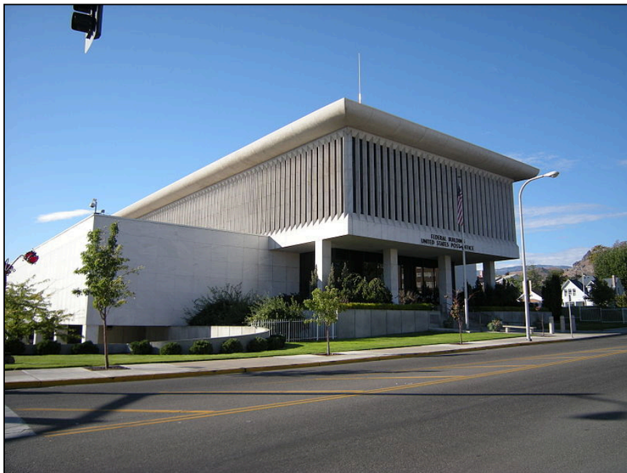
Figure 12. The Federal Building, 2008. Source: Joe Mabel, https://commons.wikimedia.org/wiki/File:Wenatchee,_WA_-_Federal_Building_03.jpg , 2008.
