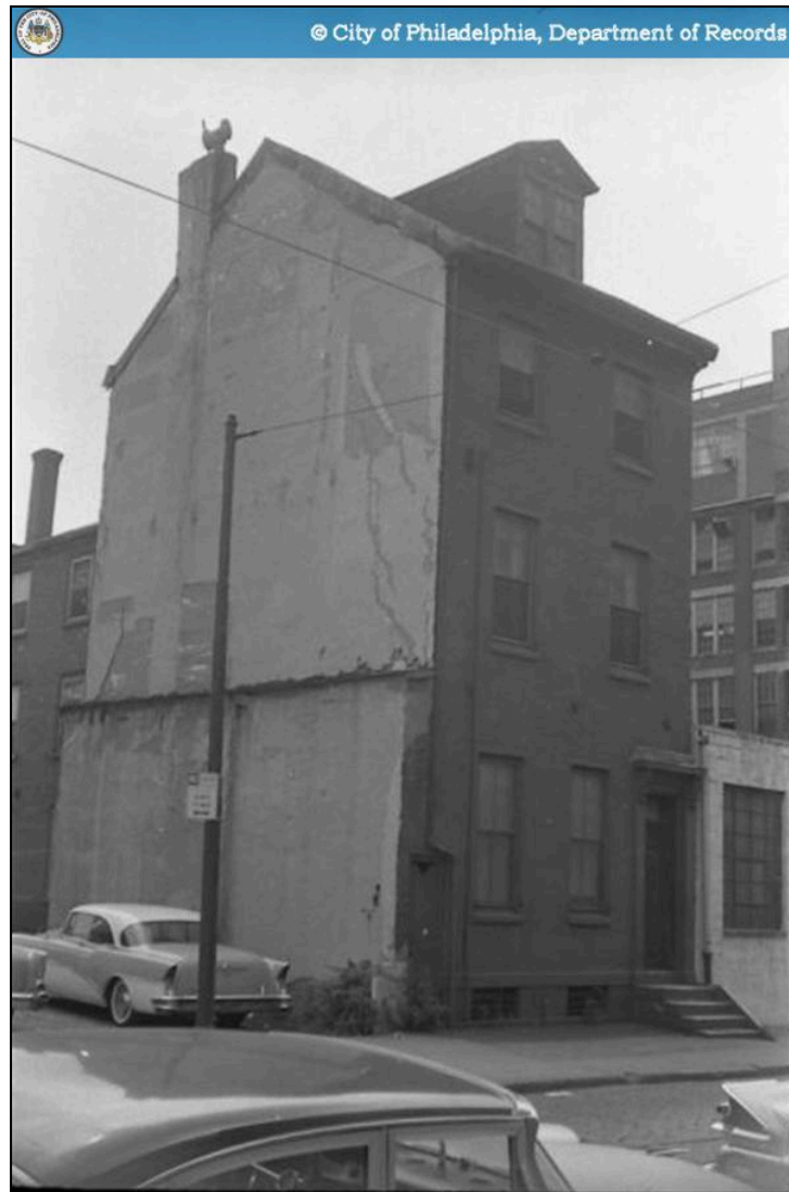
Figure 15. Looking NW at subject property in 1964 American Stores Warehouse seen in background. Source: City of Philadelphia, Department of Records, 2025.
