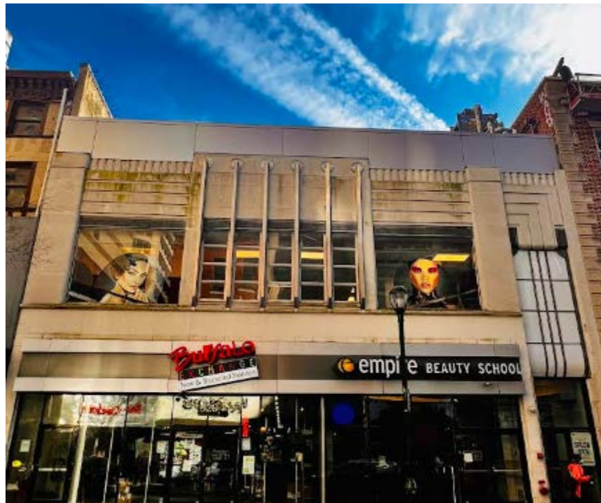
Figure 1: The primary (north) elevation of the subject property. Source: Oscar Beisert, 2022.
