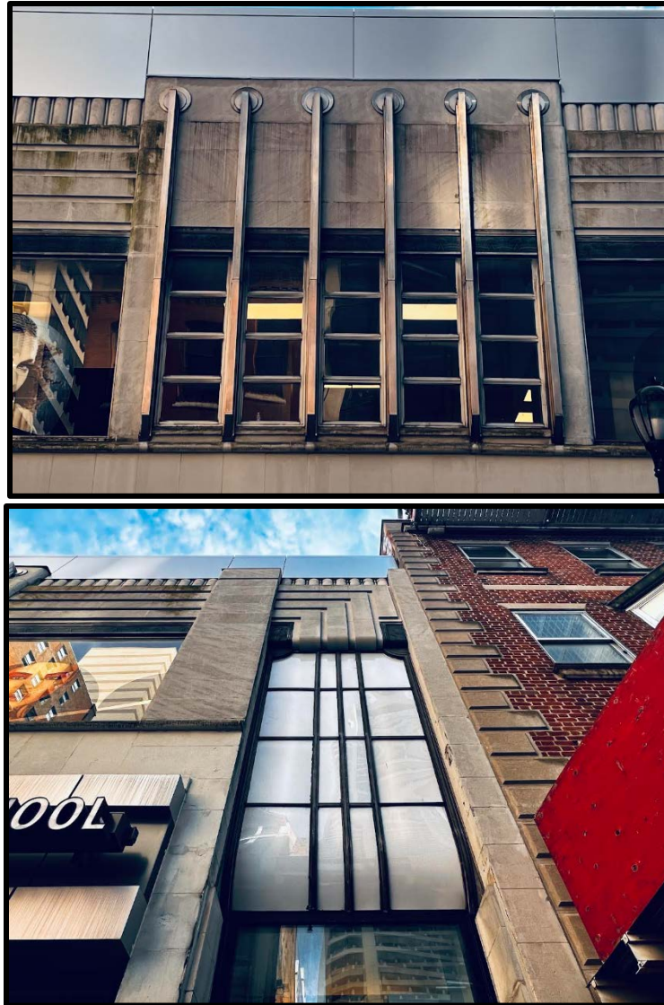
Figure 4. Top: The transom set defined by a ziggurat motif. Figure 5. Bottom: The transom's ziggurat motif and its continuation into the second floor of the primary (north) elevation. Source: Oscar Beisert, 2022.
