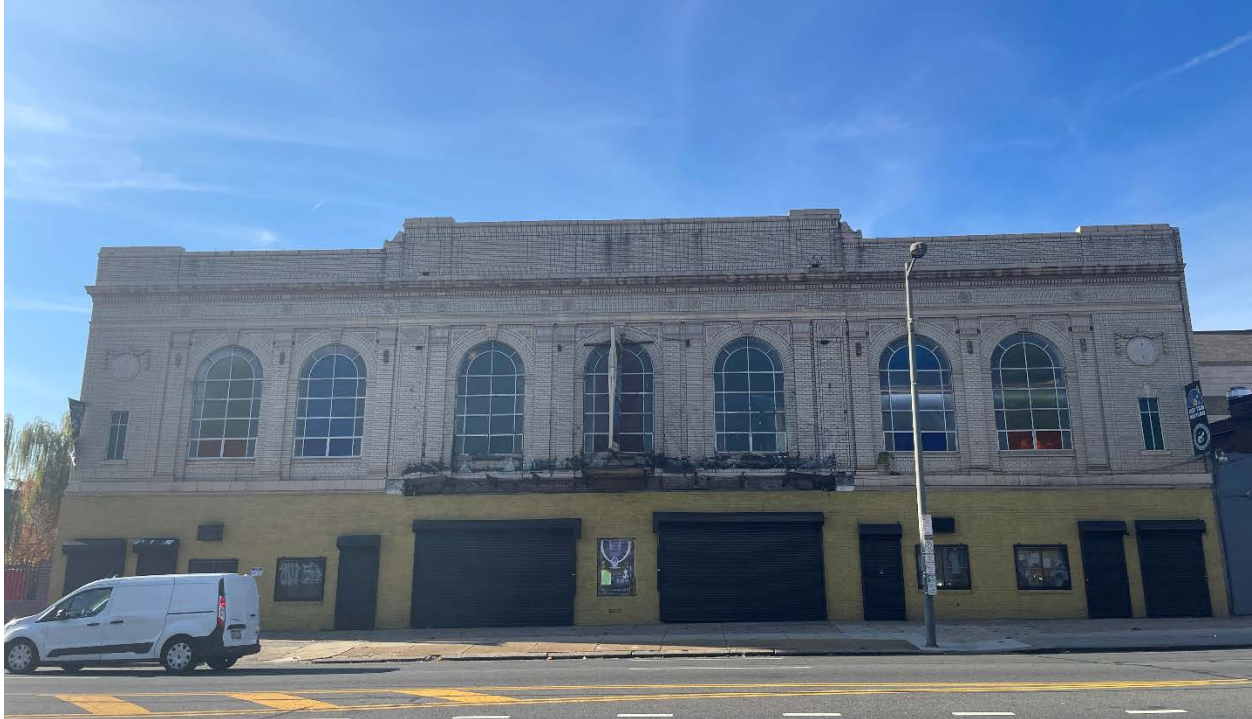
Figure 4. The primary elevation, along the west side of North Broad Street. Site photos by author, 2024, unless otherwise noted.
