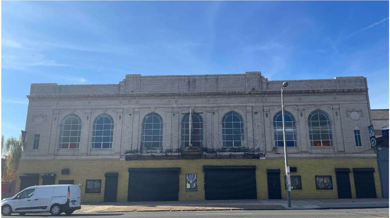
Figure 1. The primary elevation, along the west side of North Broad Street.
