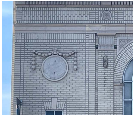
Figure 8: A large medallion appears at each end of the elevation.
