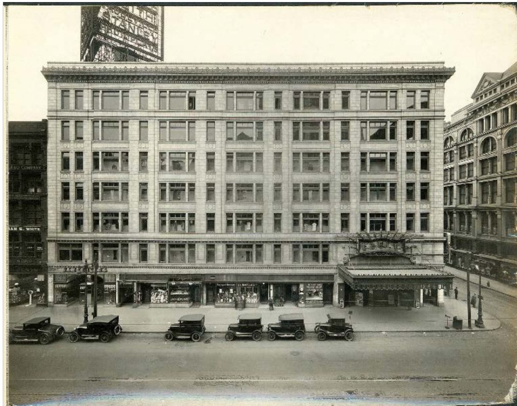
Figure 34: Earle Theatre at 11 th and Market Streets, built 1924, demolished 1953. Photo from the Glazer Theater Collection.
