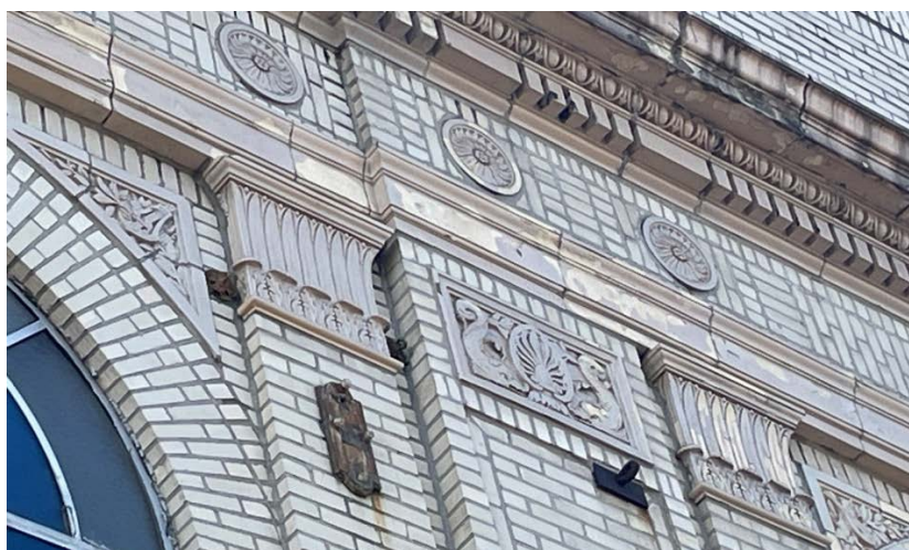
Figure 6: Capitals of the Tower of the Winds Order—small acanthus leaves with longer, flat leaves behind—top the pilasters. Botanical motifs fill the spandrels around the arched windows. The piers which set off the central section of the elevation feature palmettes in relief. Rosettes on the frieze follow the rhythm of pilasters and piers.
