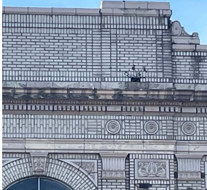
Figure 7: The keystones above the large windows also feature acanthus leaves. A volute (at top right) adorns the parapet wall. Brick laid in a variety of bonds gives visual texture to the façade.
