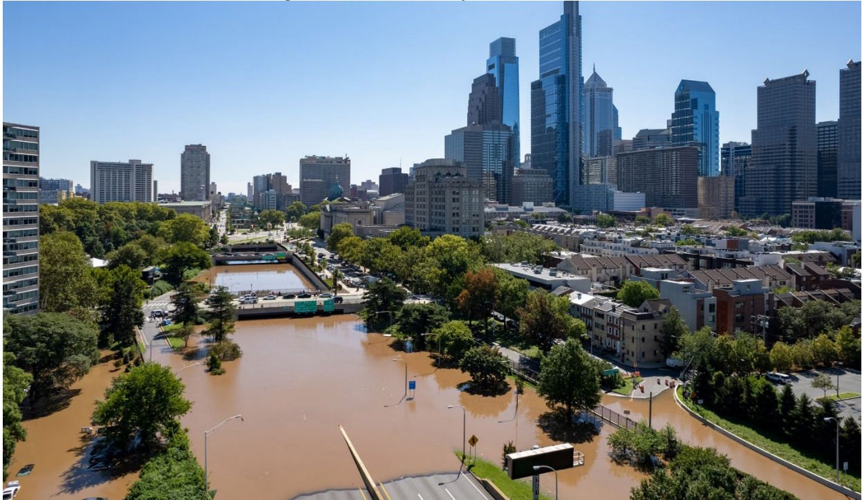
Figure 17: Interstate 676 after Hurricane Ida
