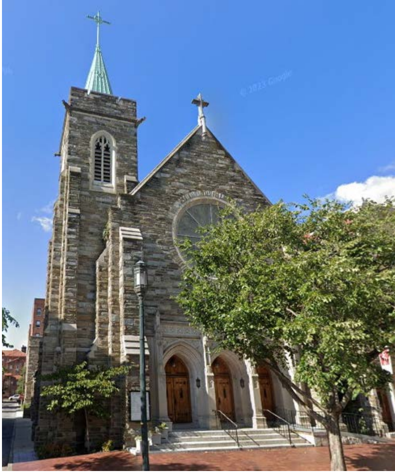
Figure 65. St. Lawrence Church, Harrisburg, PA. Paul Monaghan, Architect, 1918. Source: Google Streetview.
