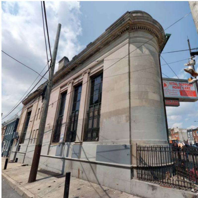
Figure 3. Potter Street facade 820-26 E. Allegheny Avenue, August 2024. Source: Cyclomedia.
