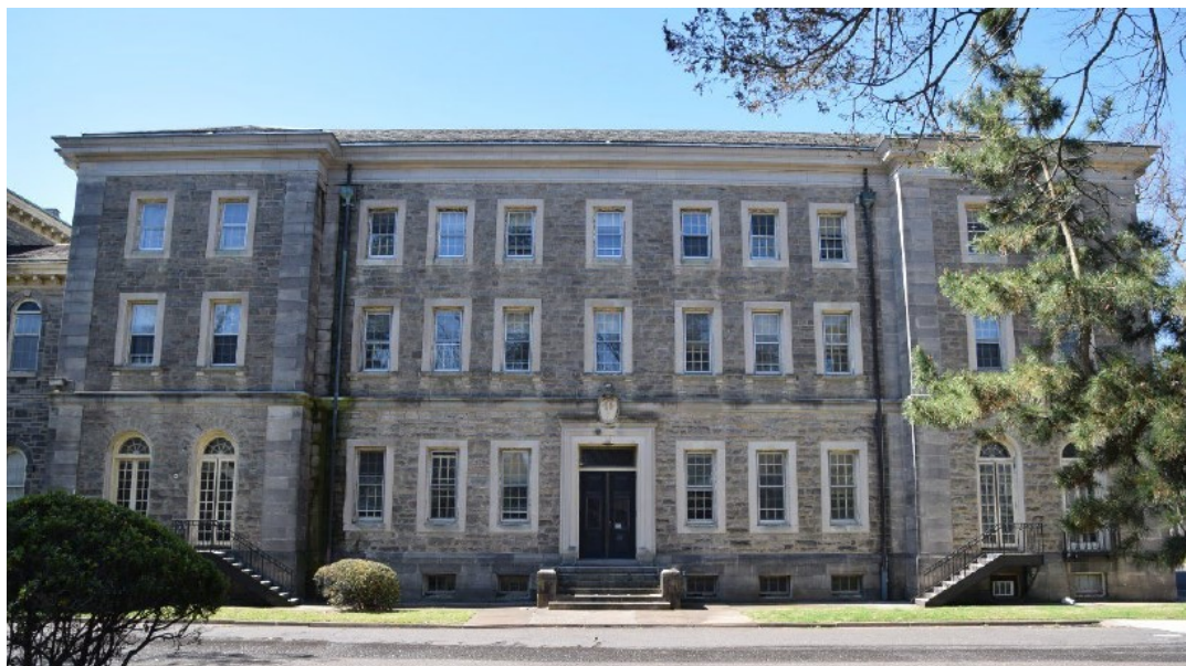
Figure 48. Service Wing/St. Neimann Hall, Paul Monaghan, Architect 1917. Source: Determination of Eligibility for St. Charles Borromeo Seminary, 2023. Source: PA Share.
