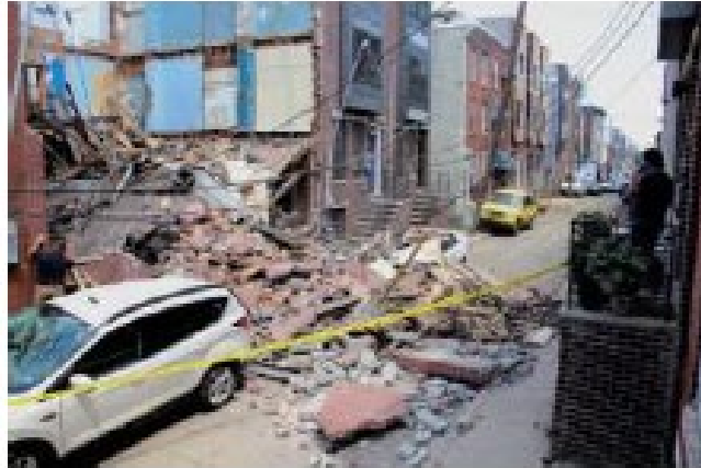
'It felt like an earthquake': South Philly rowhouse collapse crushes two cars
