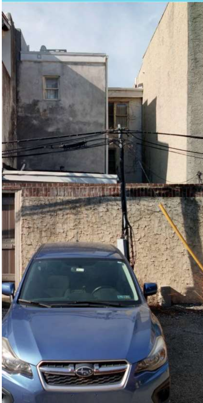
Figure 2. 613 S. Hancock Street, (Rear) 2021. Source: Cyclomedia.phila.gov
