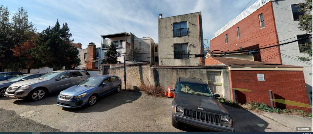
Figure 3. West Side 600 Block S. Howard Street, 2021. Source: Cyclomedia.phila.gov
