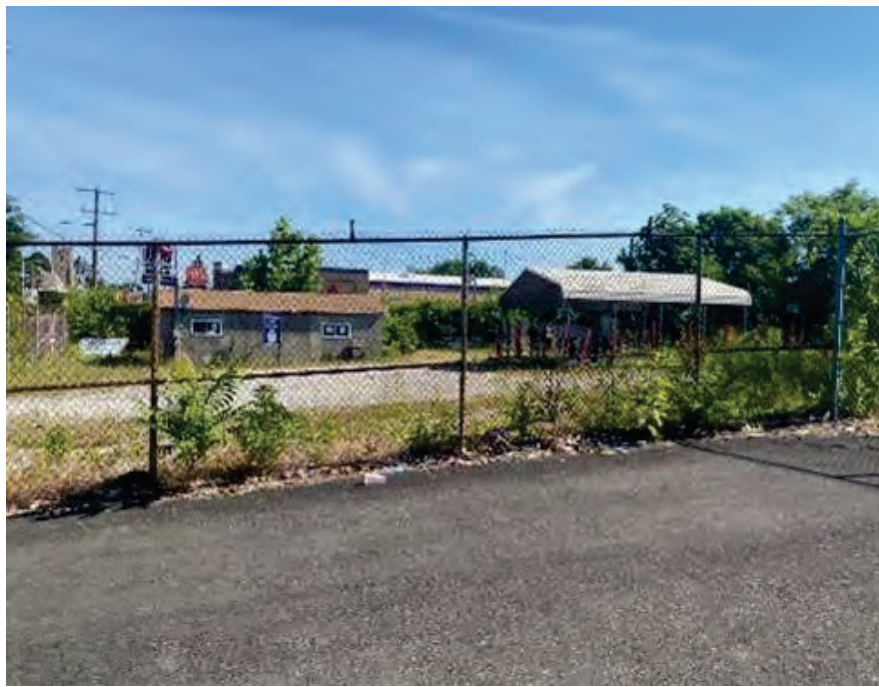
22 VIEW OF EXISTING NORTHEAST PROPANE FROM OXFORD NOT TO SCALE
