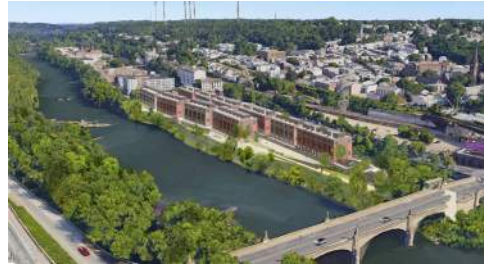
The Locks Riverside Way (1 Leverington Avenue), Philadelphia 5 Stories - 63 Townhomes
