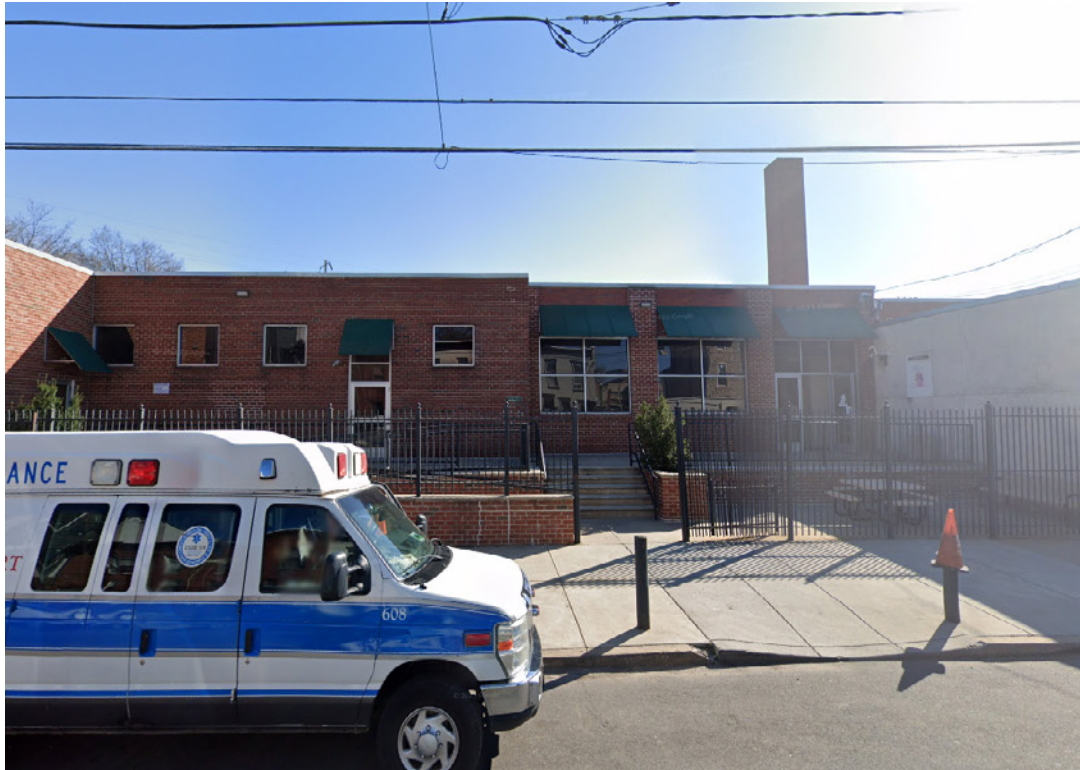
1 View from West Clearfield Street
