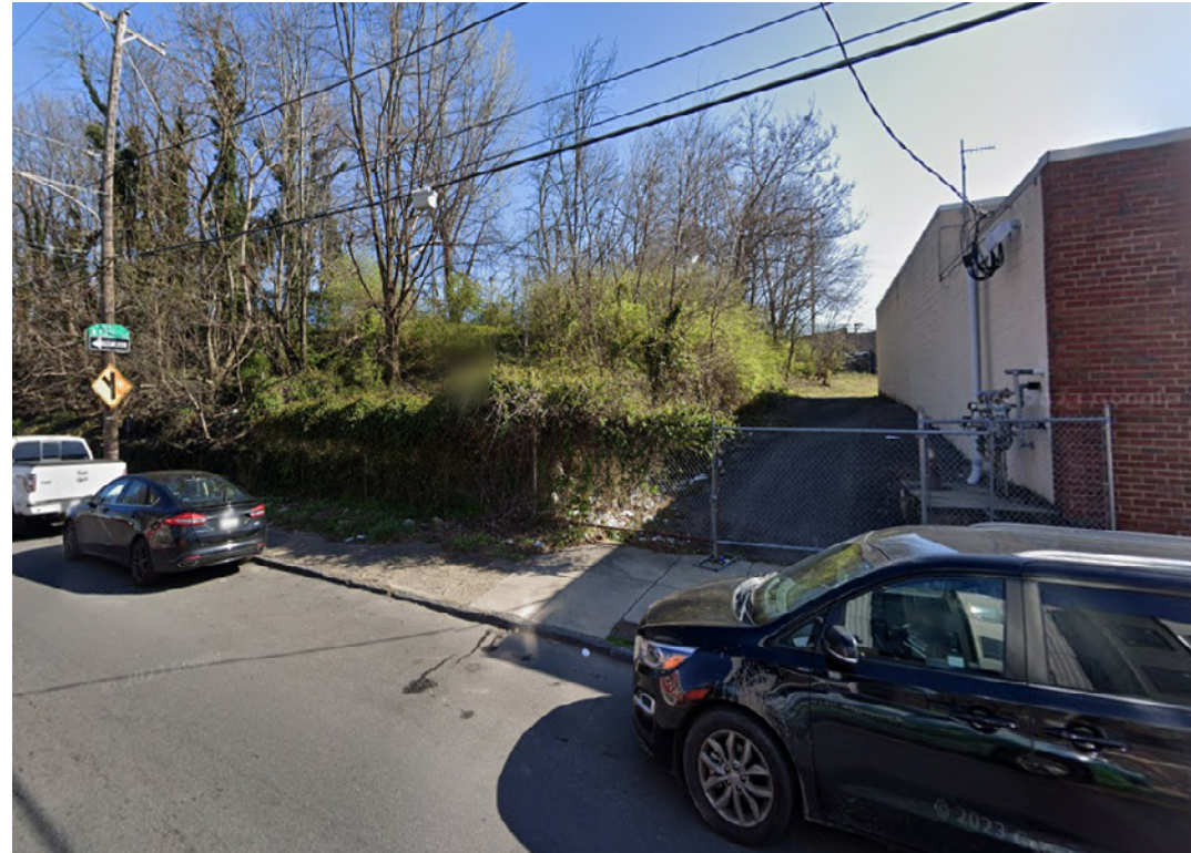
2 View of East side of site along West Clearfield Street
