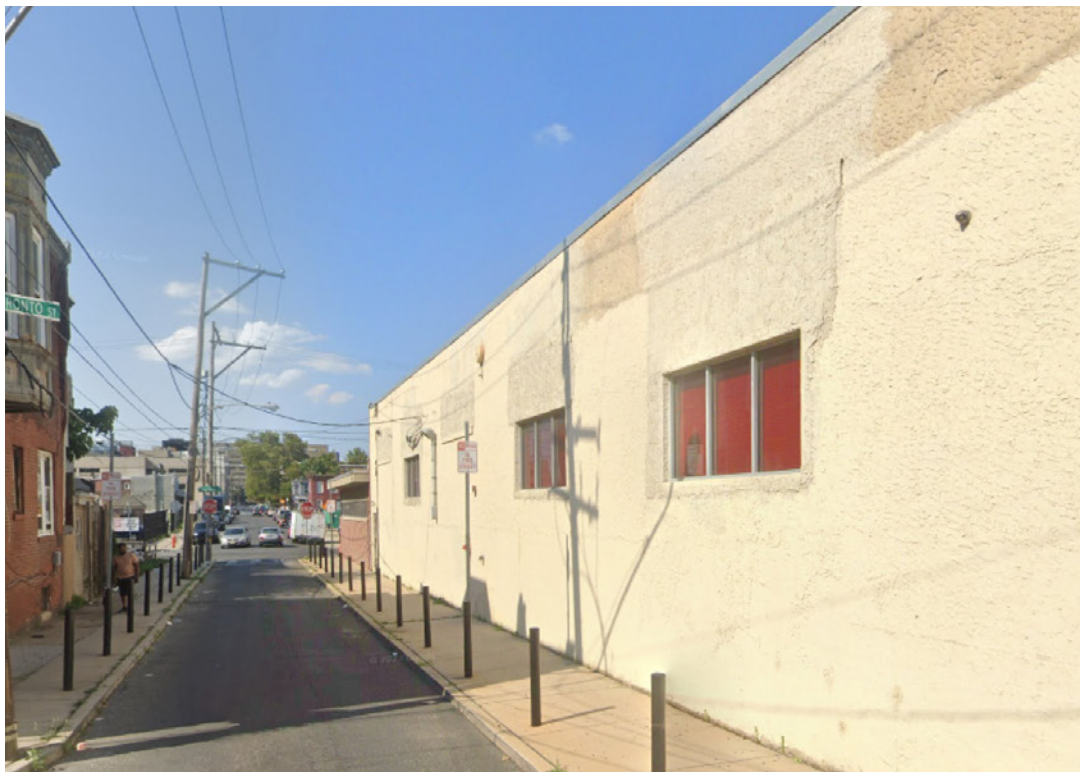
3 West side of site, looking North along Park Avenue
