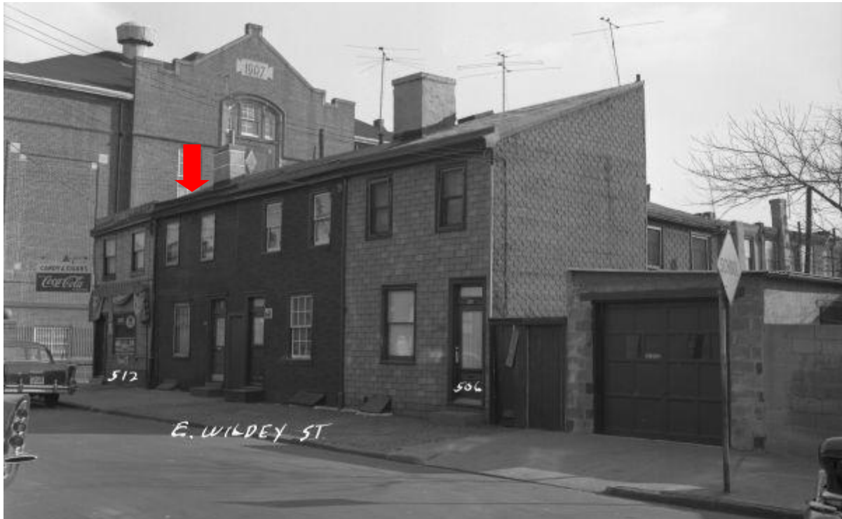
Figure 1: The row of four frame buildings on E. Wildey Street in 1958. Source: Historical Commission files.
