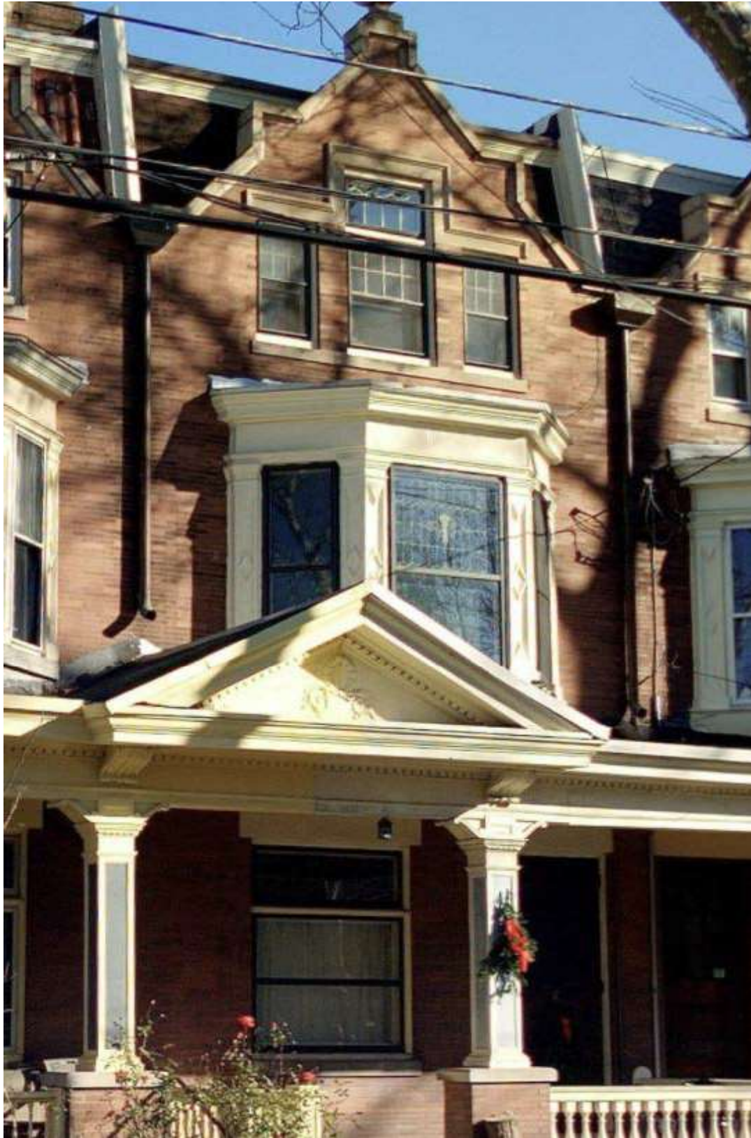
Figure 1. 327 N 34 th Street, 2021. Front windows prior to replacement. Image source: Cyclomedia.
