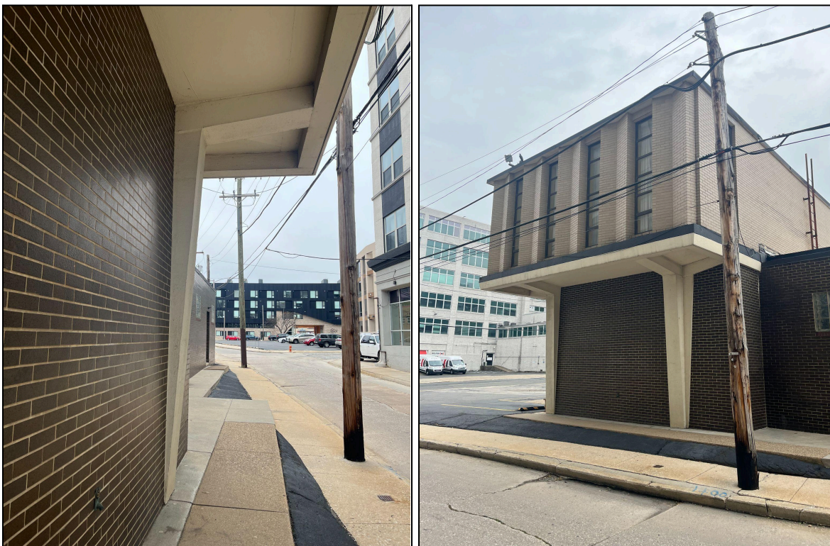
Figure 3 and 4. Details of Northern elevation of subject property. Source: Misha Wyllie, 2024
