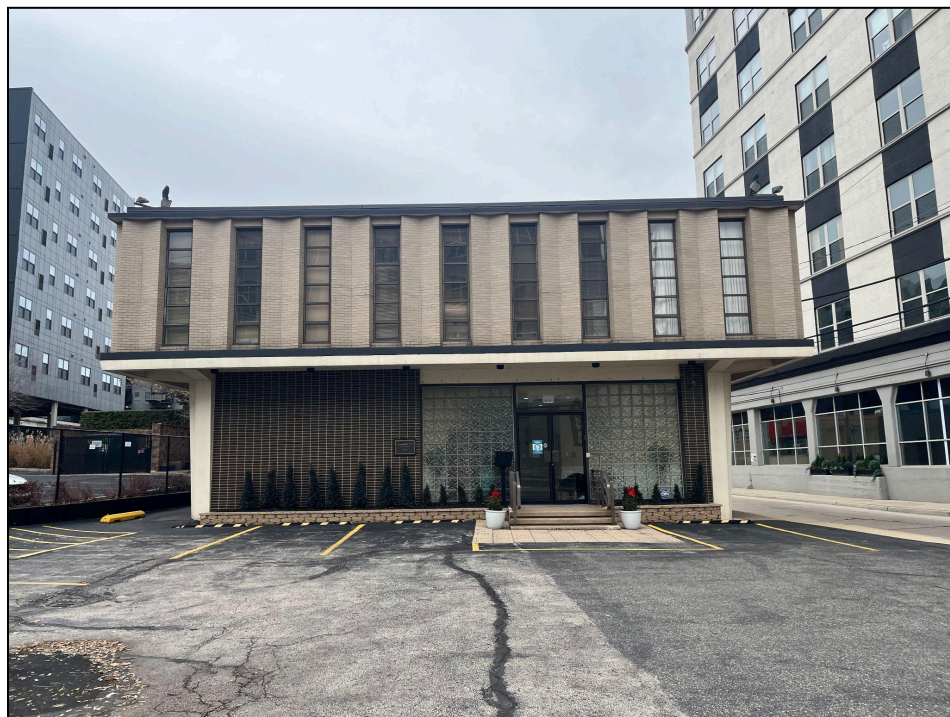
Figure 25. NMEBA Front, Eastern Elevation. Source: Misha Wyllie, 2025.
