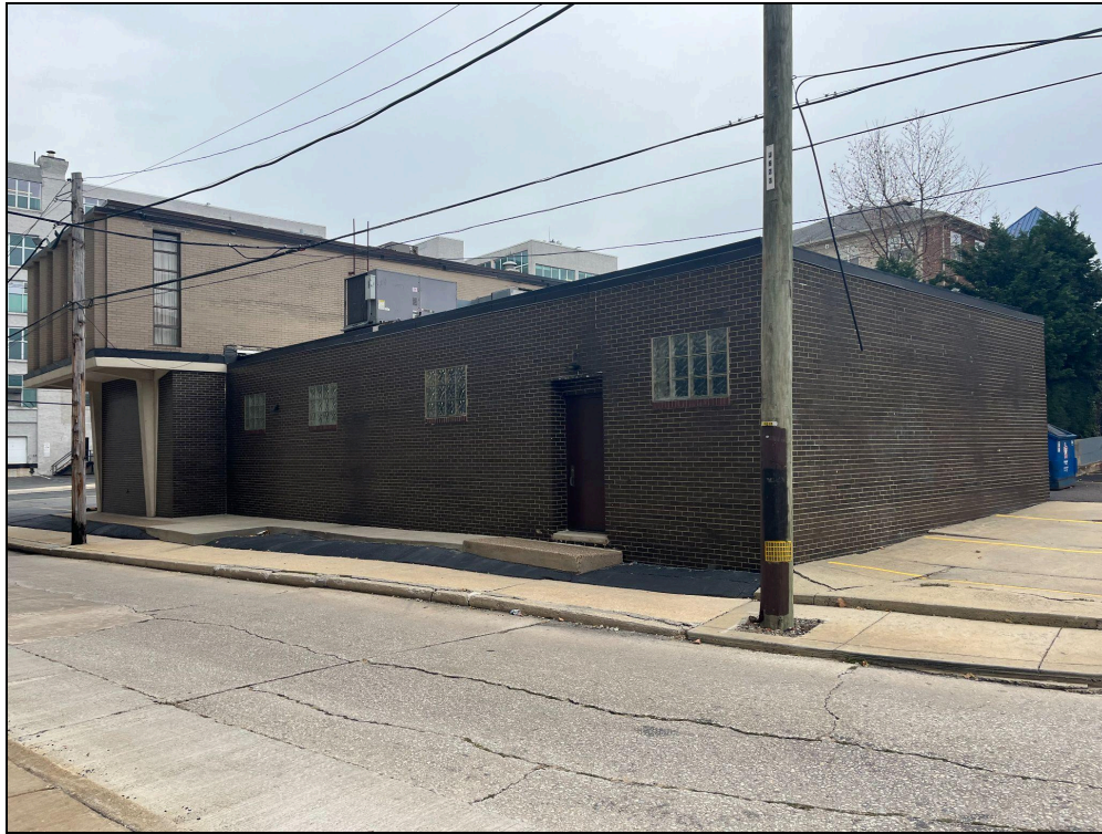
Figure 5. Northern and Western elevations of subject property. Source: Misha Wyllie, 2024.
