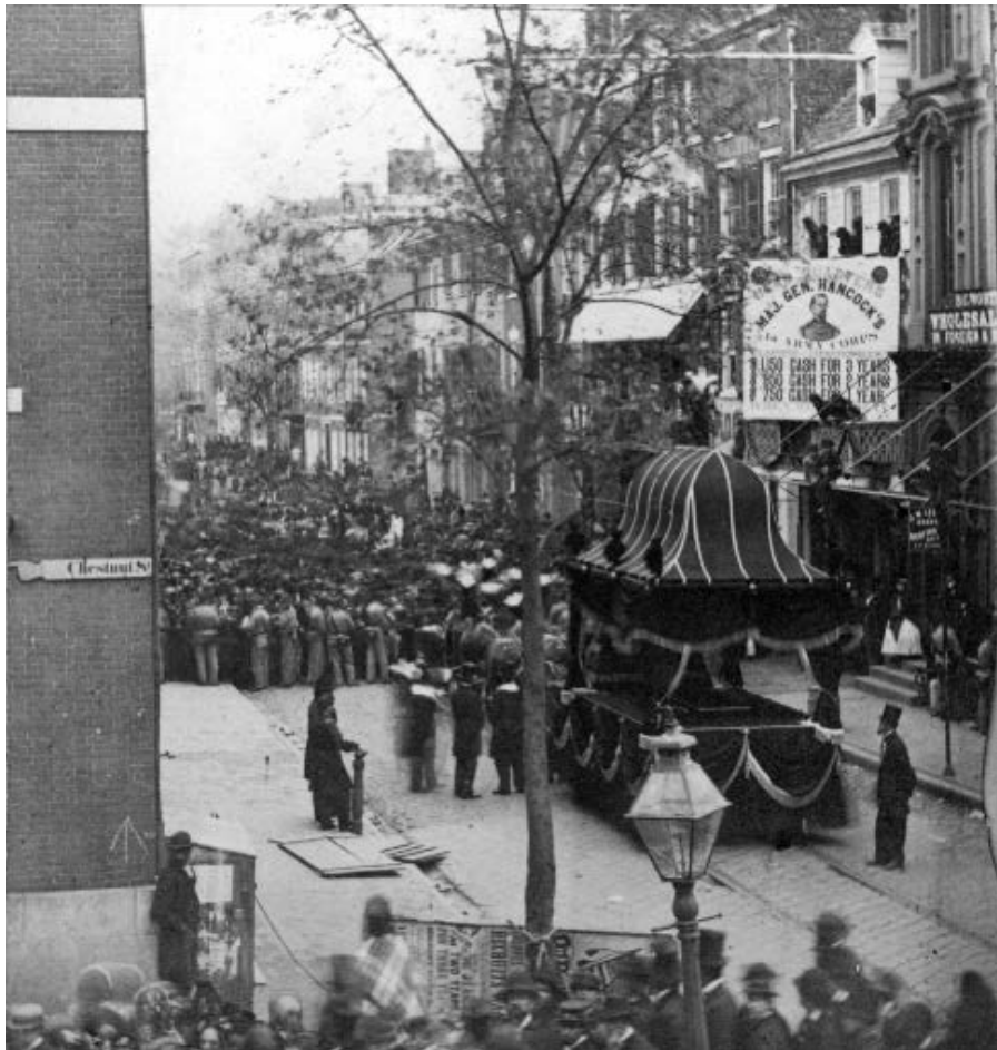
Figure 32. A photograph of Lincoln's hearse stopped on S. 6 th Street, facing south, on April 22 or 23, 1865. The building on the left is Congress Hall, which is to the west of Independence Hall. The building on the right in the foreground houses B.C. Worthington, wholesale dealer in foreign and domestic segars, located at 102 S. 6 th Street, as noted in the McElroy's City Directory of 1865. Ridgway Glover, photographer. Source: Huntington Digital Library.
