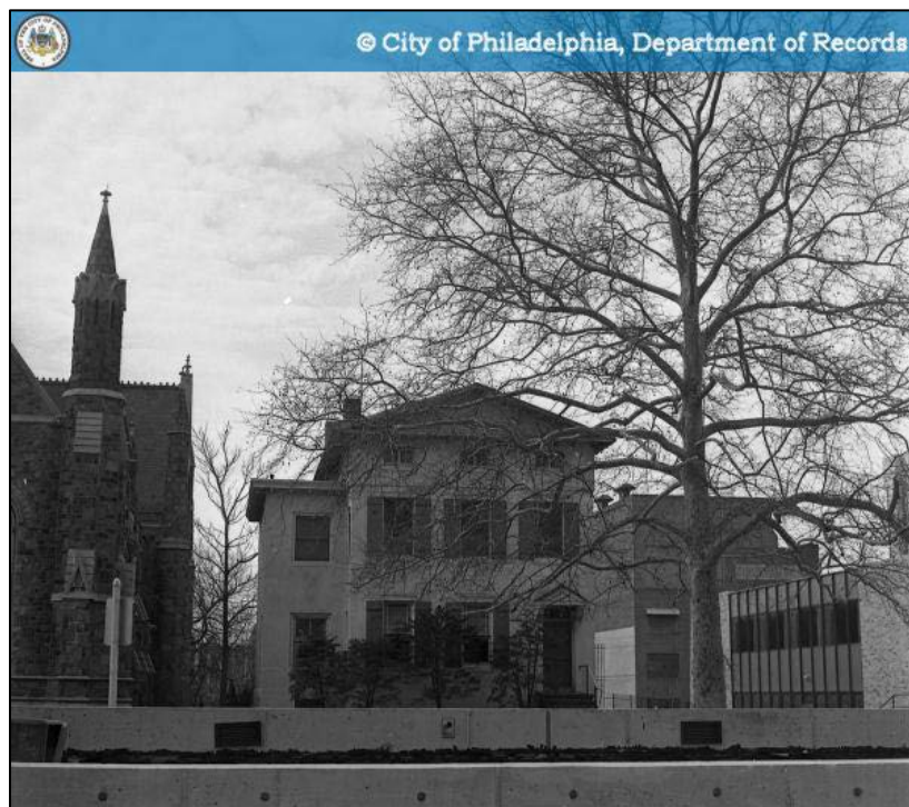
Fig. 12. Photograph dated 1971 showing window shutters at north elevation. Source: City of Philadelphia, Department of Records.
