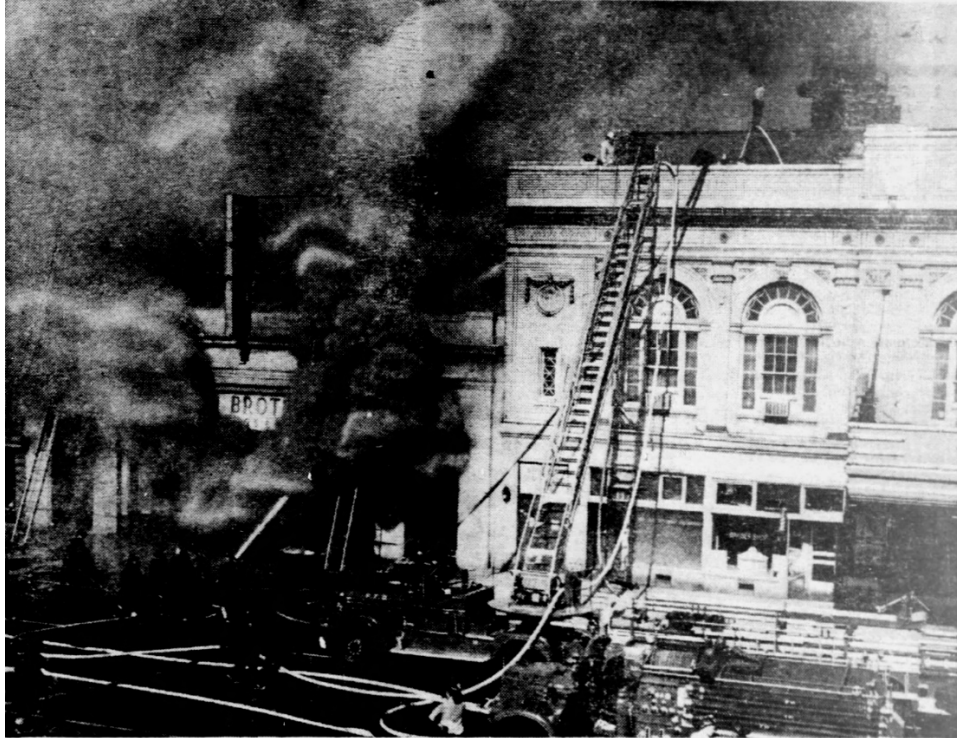
Figure 24: A 1965 newspaper photo shows the condition of the Logan Theatre during a fire to the neighboring building, now demolished. The original pane arrangements of two storefronts can be seen after the removal of their awnings. The center portions of the fan lights on the second floor appear to have been replaced by solid panels. Photo from the Philadelphia Daily News , May 21, 1965.
