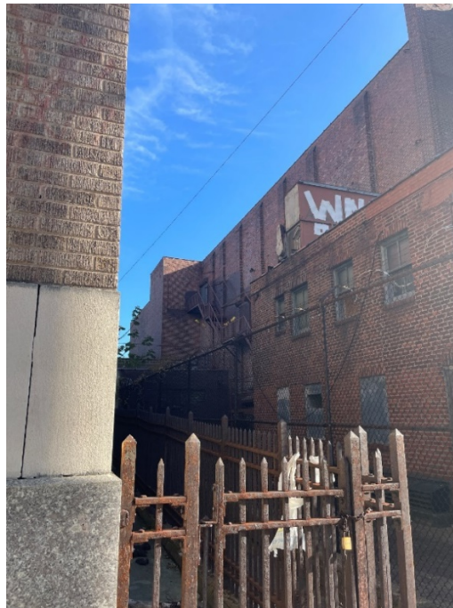
Figure 19: Oblique view of the north elevation of subject property, seen from Carlisle Street. The free-standing utility building can be seen to the left and the former Dressing Rooms structure is at right.
